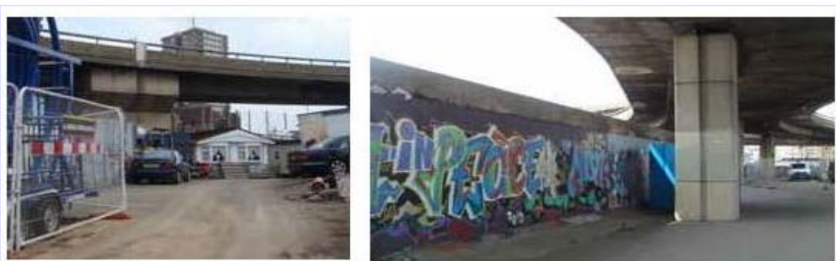
Figure 4 Stable Way and Westway Sports Centre - Issues
