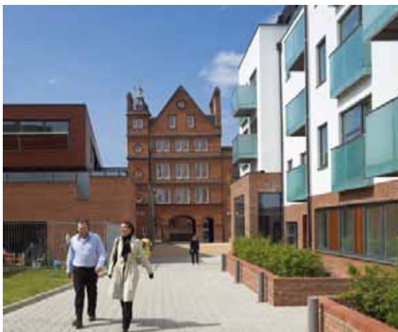
Existing view to the Harrow Club (right) and a new development which respects the setting of a similar character building (left) HORNSEY ROAD, POLLARD THOMAS EDWARDS
