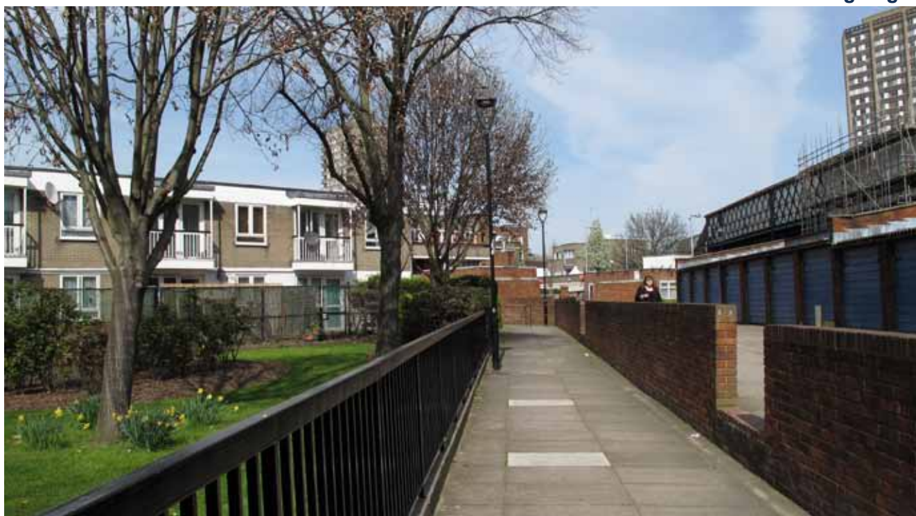
Footpath in front of the garages
