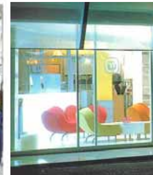
Sections of existing arcade replaced by glazing
