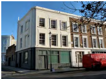
Here is Penzance Place , followed by 12A Penzance Place, and the backs of houses in Pottery Lane, all in keeping with the 1840's architectural patterns. (The numbering here is discontinuous, which may indicate that the backs of the houses now in Pottery Lane were once numbered as in Princedale Road.)
