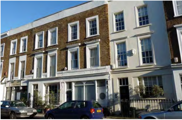
54-60 Princesdale Road. It would be desirable to reinstate the original window designs.
