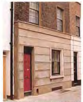
Middleton Buildings: Successfully detailed and finished reinstatement of band-rusticated stucco.
