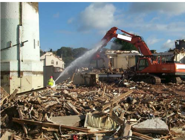
Figure 3 Damping down of demolition materials before handling
