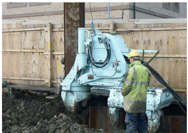
Figure 10 Hydraulic piling is a relatively quiet piling method
