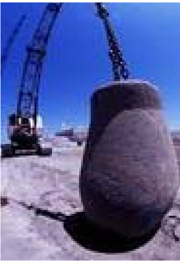
Figure 5 A demolition ball in action
