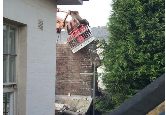
Figure 6 Grab attachment fitted to an excavator
