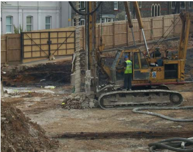
Figure 11 Auger piling for building foundations
