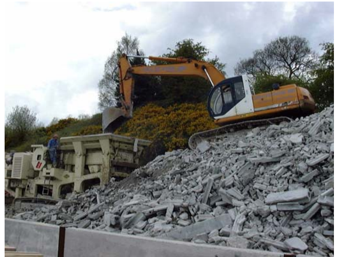
Figure 12 Crushing and grading concrete components into recycled aggregates
