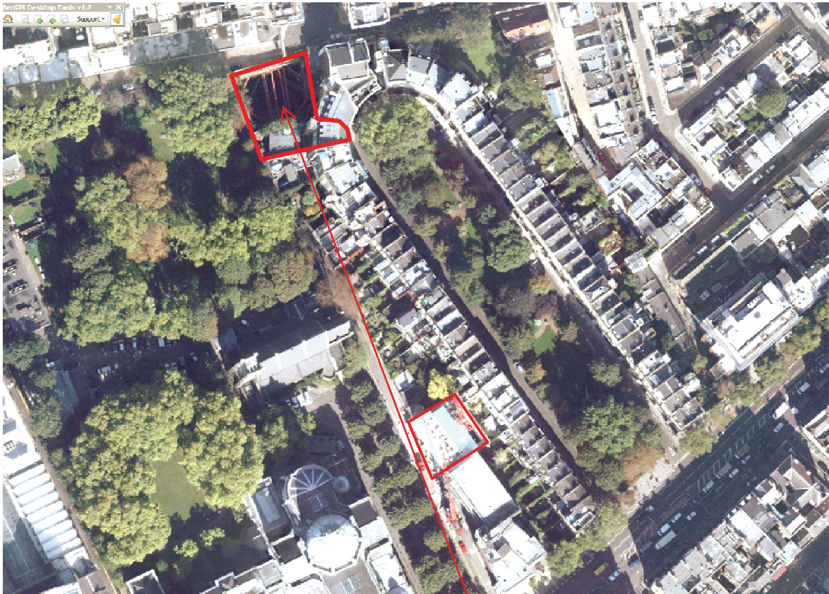
31 Brompton Square and 7-10 Cottage Place 2011 (Note the excavation at 31 Brompton Square with loss of all natural permeable ground and planting)
