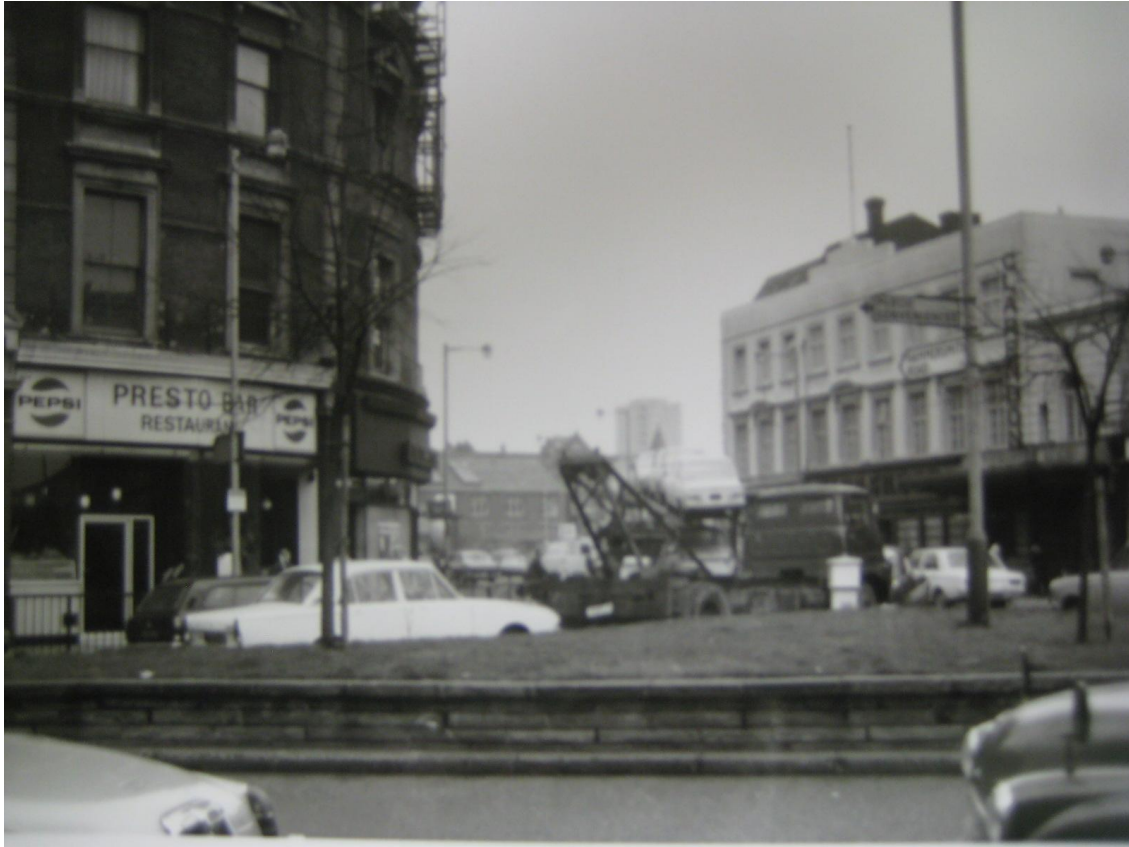
Fig.1 – Lime tree in soil filled raised planter 1971. Available soil volume estimated at 40 cubic metres.
