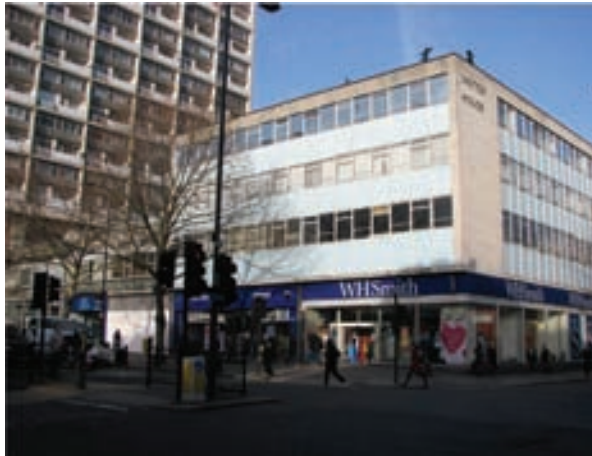
Buildings in need of renovation and repair
