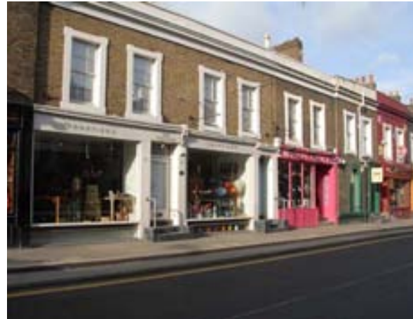
Existing shop fronts provide overlooking and animation to Pembridge Road
