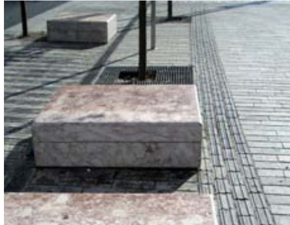
Grand Parade Cork: Natural stone blocks offer informal seating and mark the limits of parking bays
