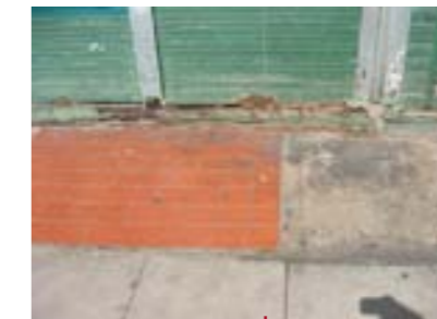
Patch pavement materials
