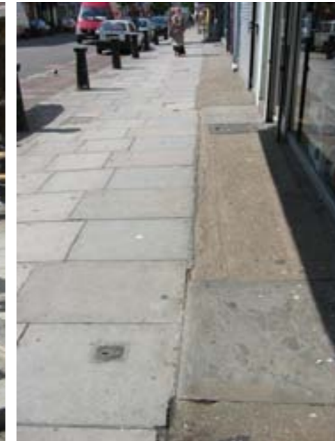
Concrete slabs and a crude concrete edge to shop frontages
