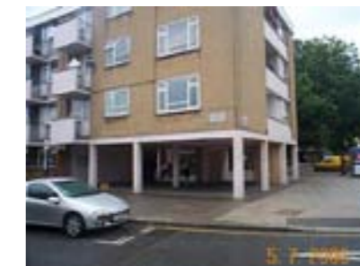
Under-used spaces beneath and alongside buildings
