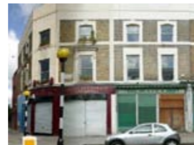
Shop units used only for storage
