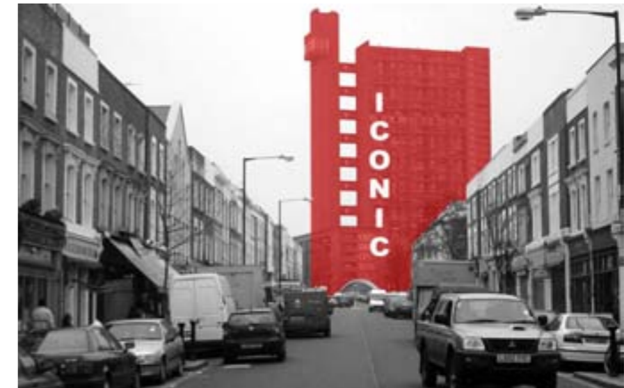
Trellick Tower is a key landmark in the local area and the wider urban environment
