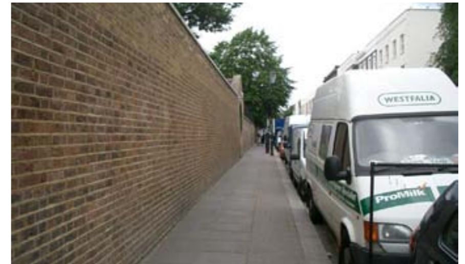
A dull brick wall creates a negative edge near the Spanish school
