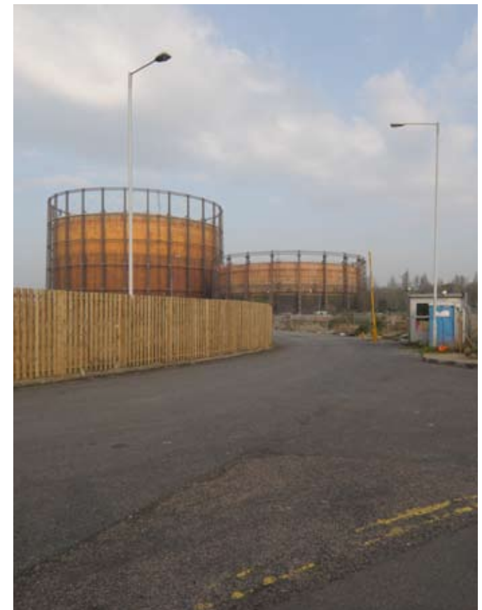
entrance to Kensal Gas Works
