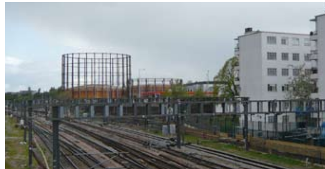
view from the railway bridge, east of the site
