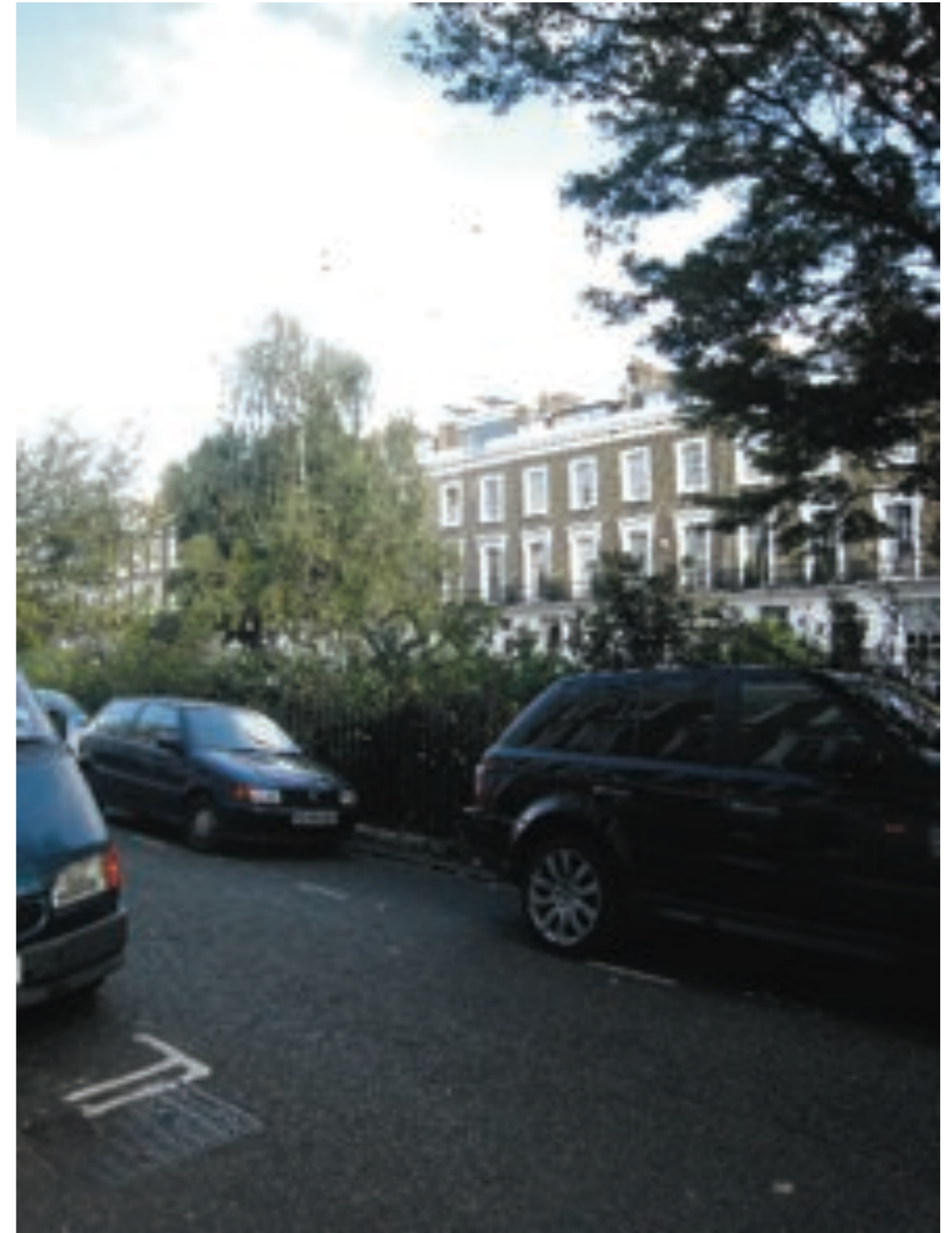
B Proposed view from South West corner of Markham Square showing PVs
