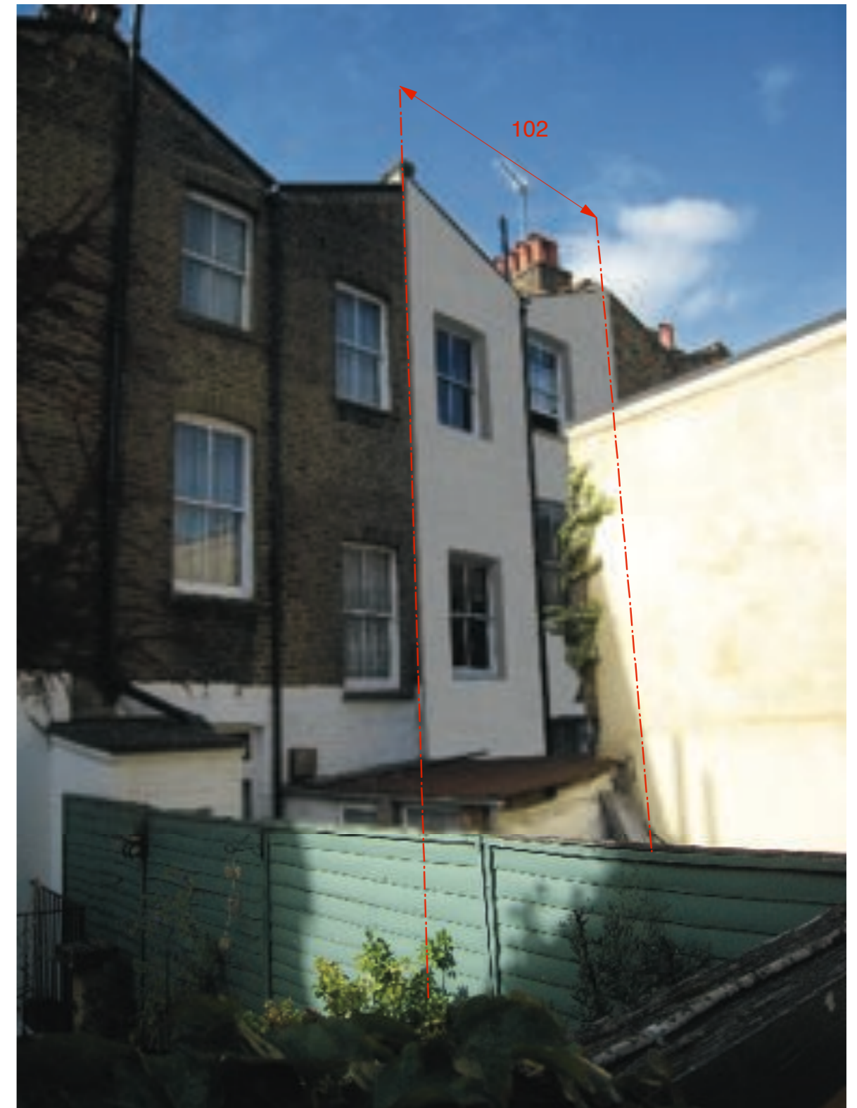
B Rear elevation externally insulated and rendered
