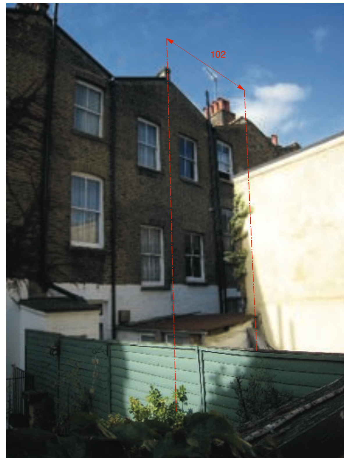
B Photo of rear elevation
