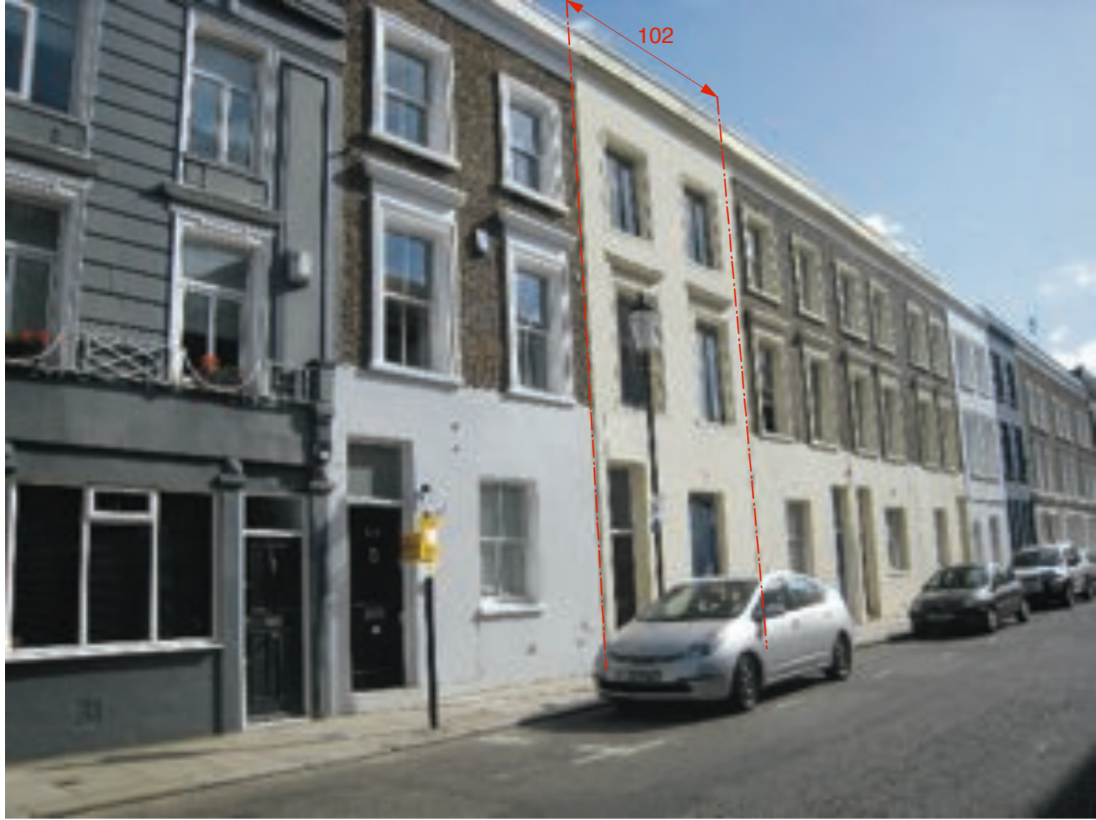
A Front elevation externally insulated and rendered, Casement windows
