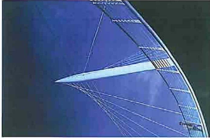
MANCHESTER CALATRAVA BRIDGE
