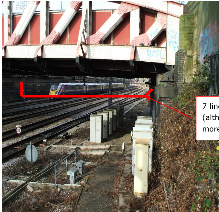
Photo 3: looking west from Goldborne Road bridge
