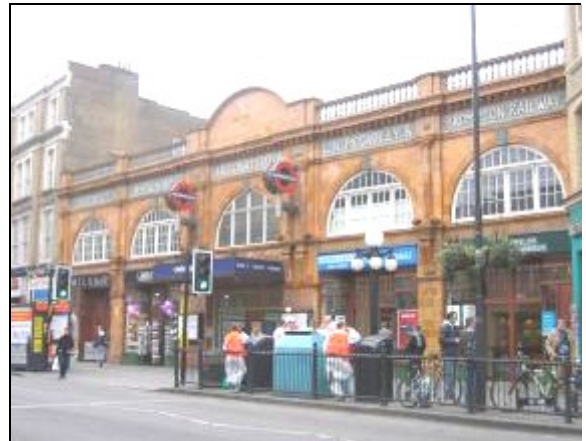
Earl's Court Road Underground Station
