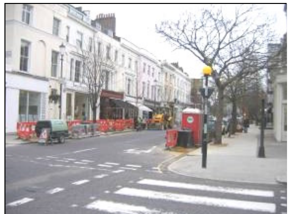
Ledbury Road Junction, with paving improvements being carried out
