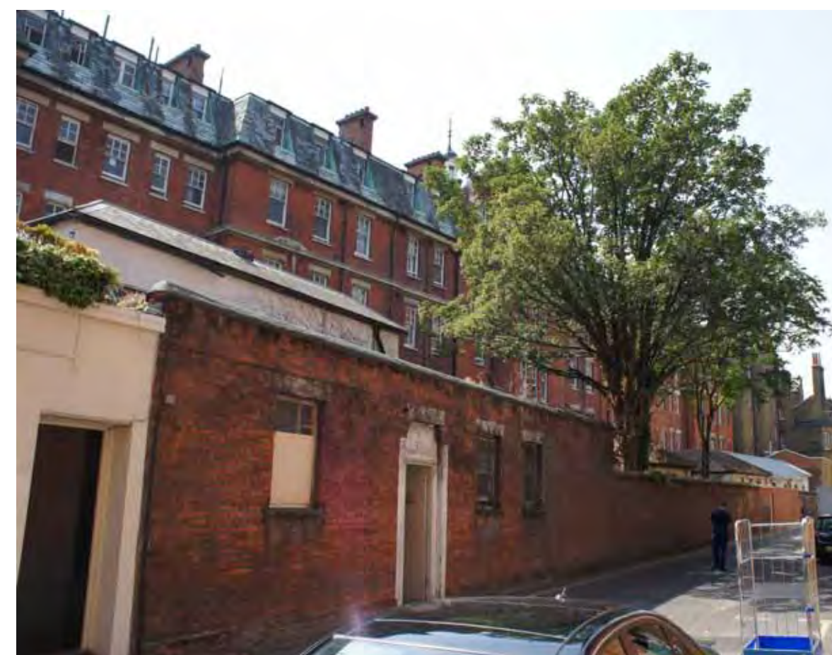
The south elevation Dudmaston Mews
