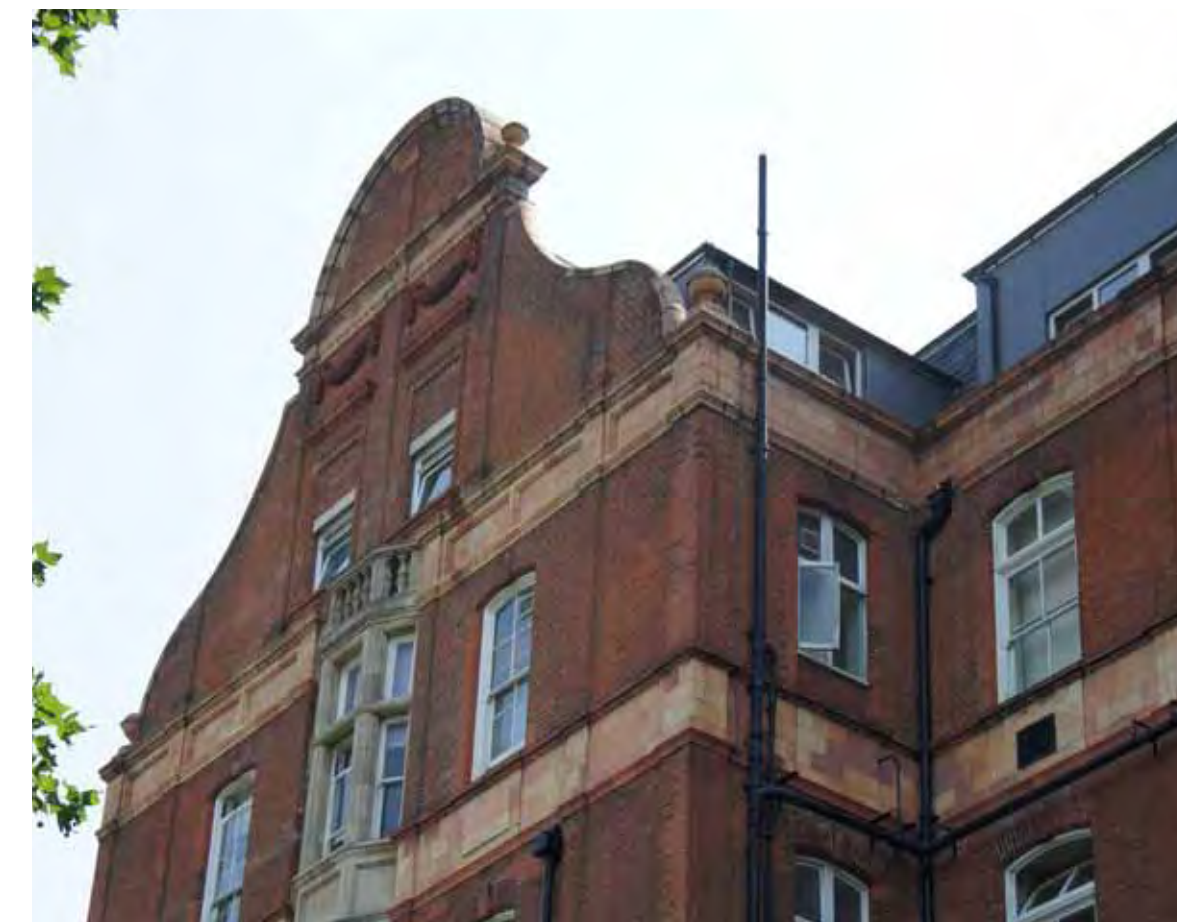
The detailing of the gables on the Fulham Wing
