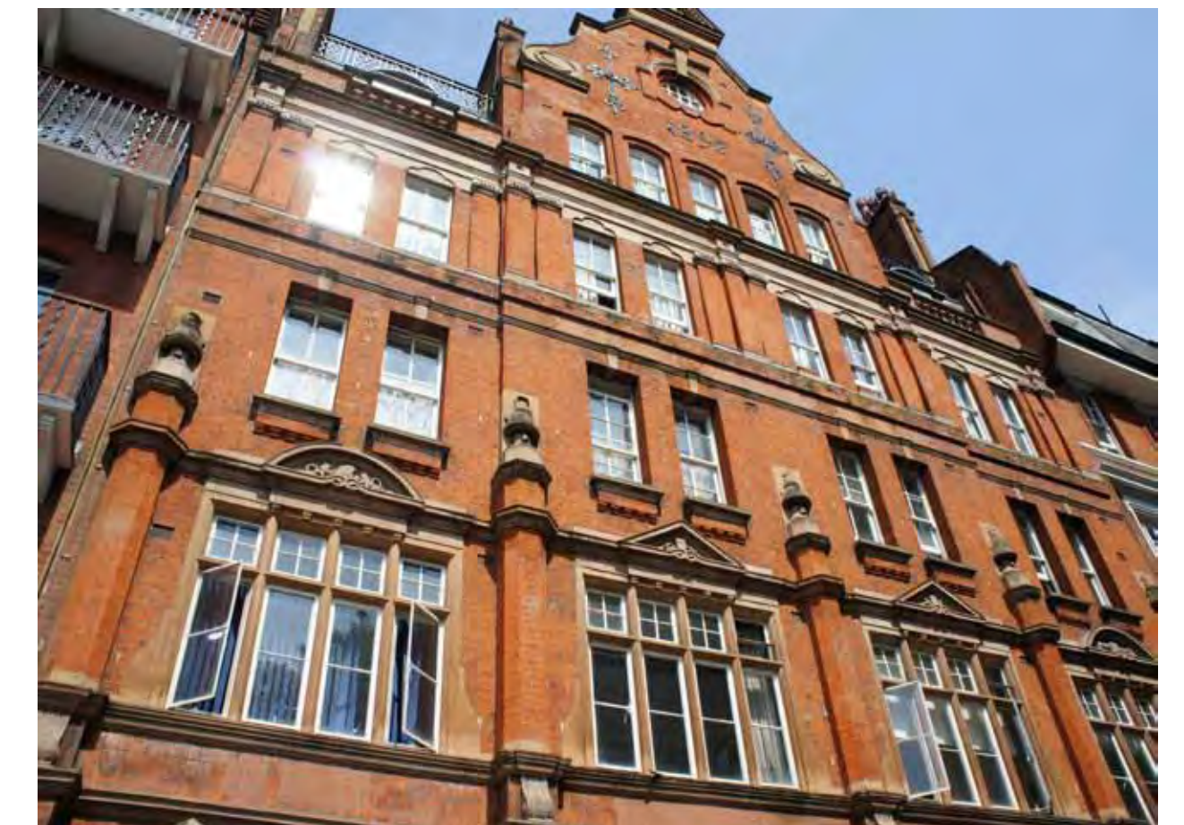
Detailing on the fire station's front elevation
