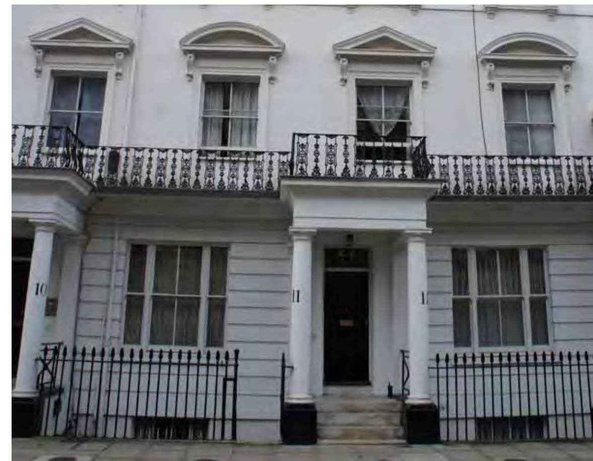
Front elevation of Foulis Terrace
