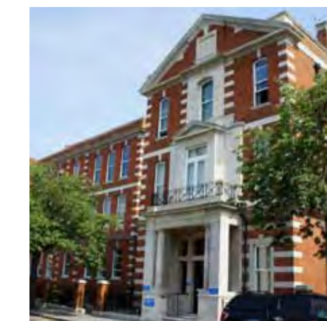
Site D: Hospital Dovehouse Street
