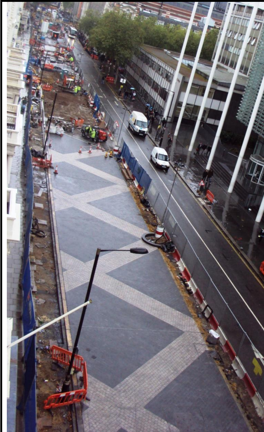
A finished section of criss cross granite paving
