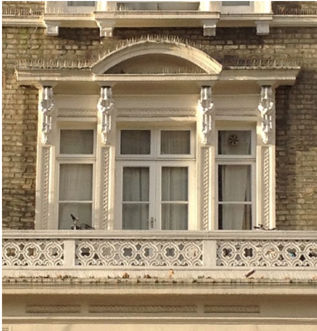
Victorian first floor feature window
