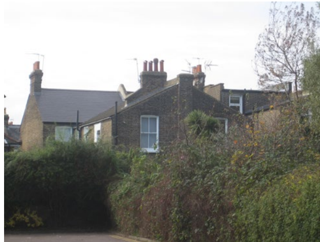
Plain pitched slate roof to main roofs and outriggers
