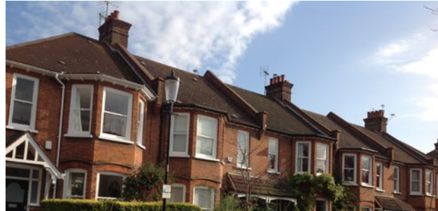
Plain pitched roofs with hipped roof terminating the terrace
