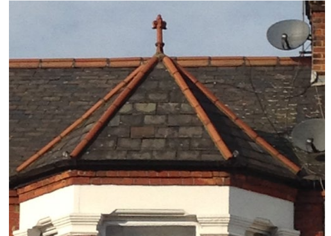
Roof finial, clay ridge and hip tiles
