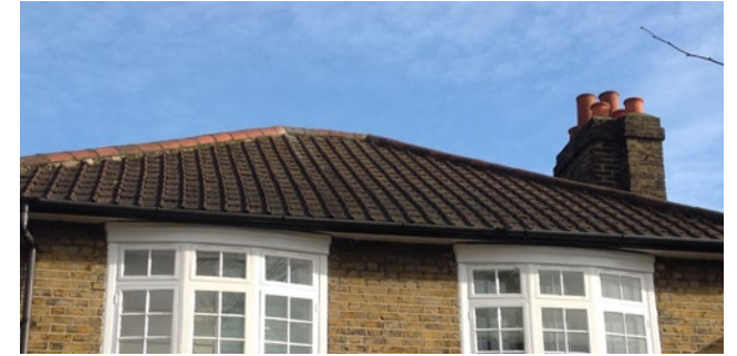
Hipped roof with original Courtrai roof tiles
