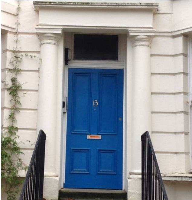
Victorian four panelled door
