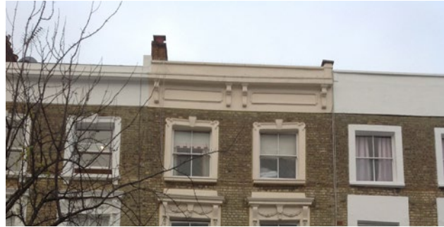
Parapet concealing butterfly roof
