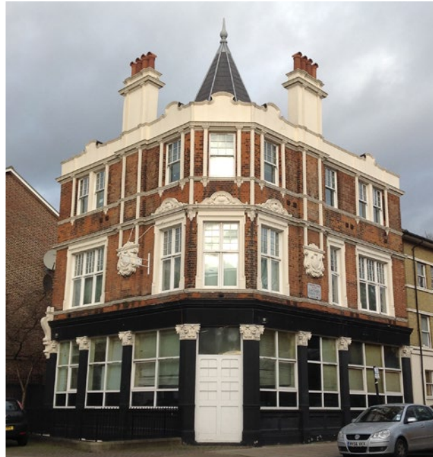
Former Public House, Latimer Road
