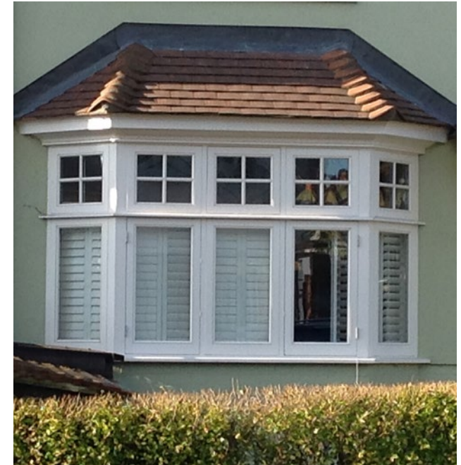
Mid 20th century casement with drip mould
