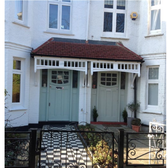
Mid 20th century doors
