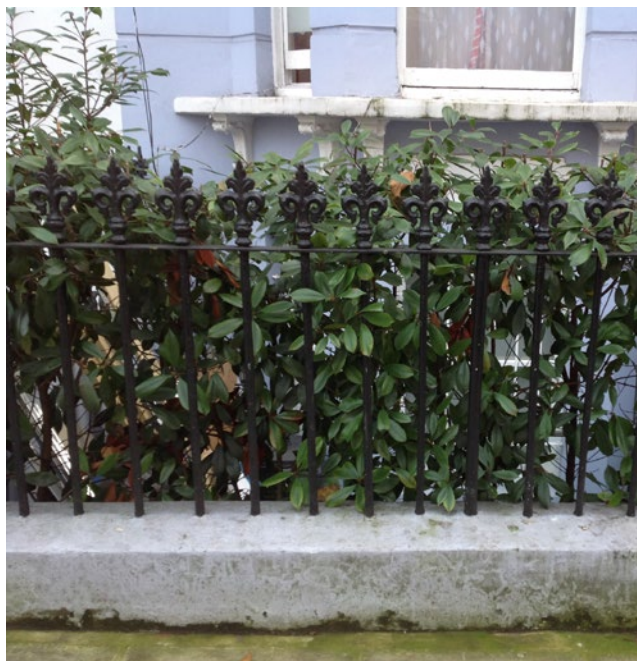
Victorian cast iron railings, Chesterton Road
