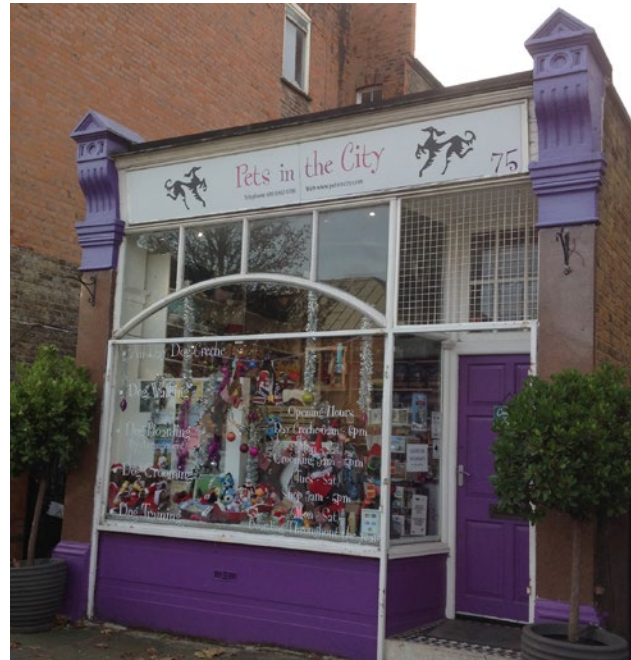
Edwardian shopfront elements, St. Helen's Gardens
