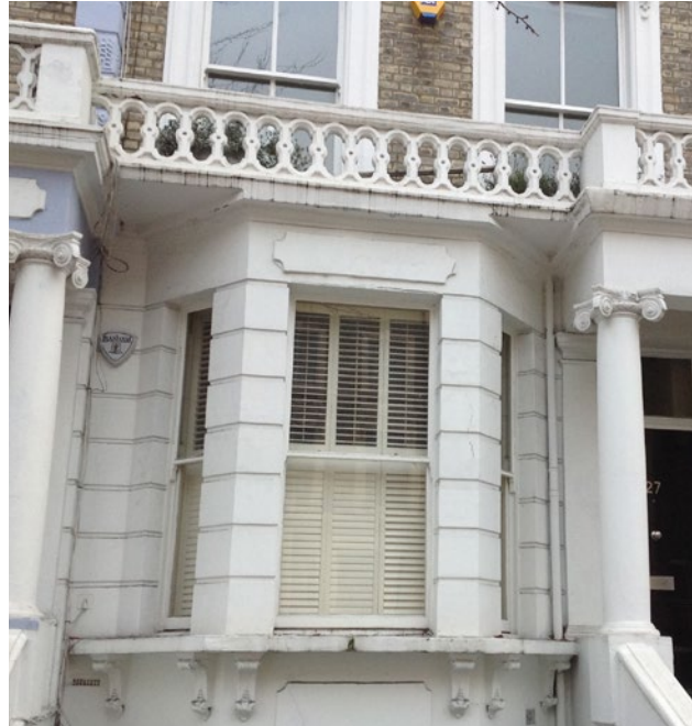
Channelled stucco with balustrade above
