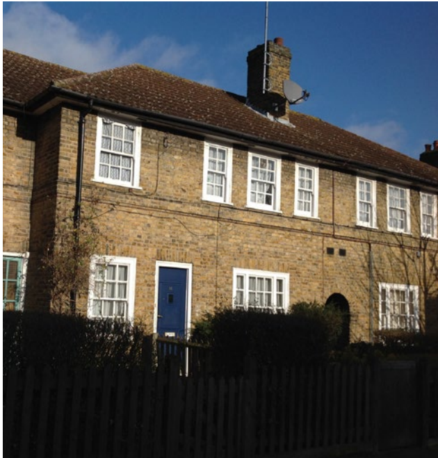
Original six-over-six sash windows
