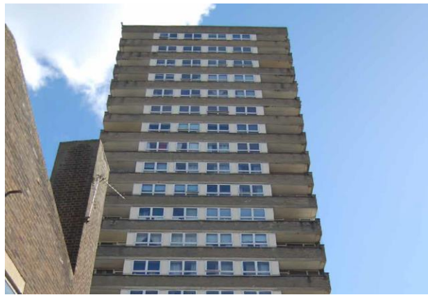
5 Whitstable House – existing RBKC residential building with landscape and parking areas
