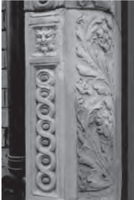
Two terracotta: the one on the left shows signs of damage and erosion following the decay of the fireskin.
