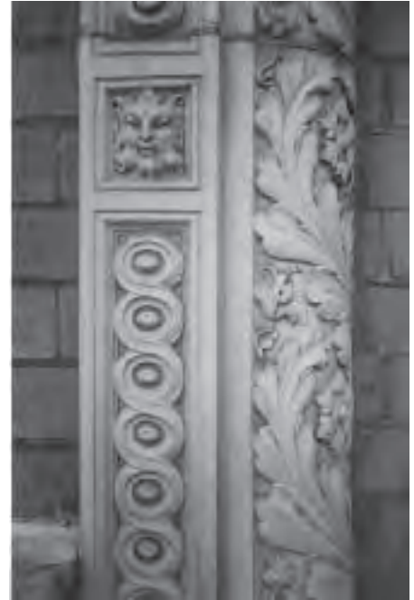
Two terracotta: the one on the left shows signs of damage and erosion following the decay of the fireskin.
