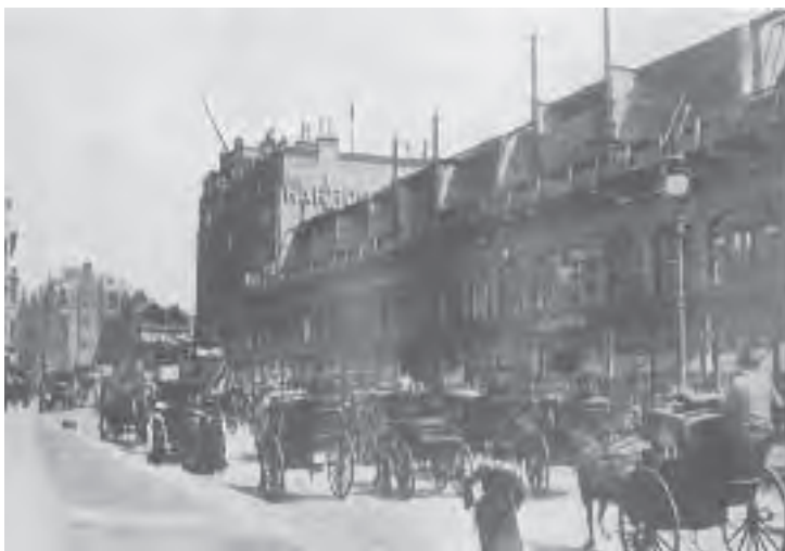
Harrods during re-building
