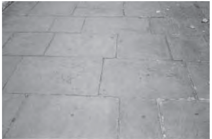
Yorkstone paving laid in courses
