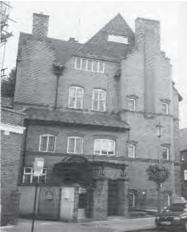
Walton House, Walton Street (Architect: R. Norman Shaw)
