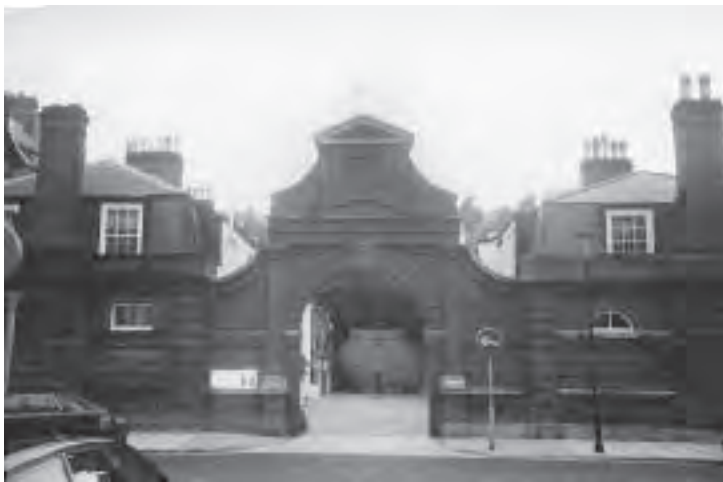
Entrance to Shafto Mews
