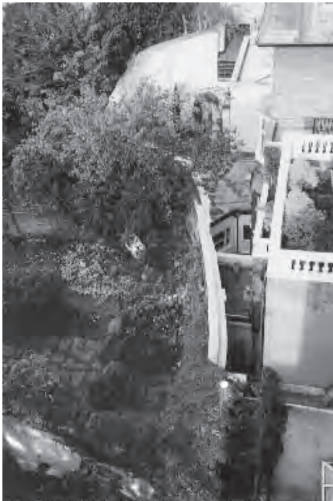
Walls denoting the course of the River Westbourne between Chesham Street and Cadogan Lane
