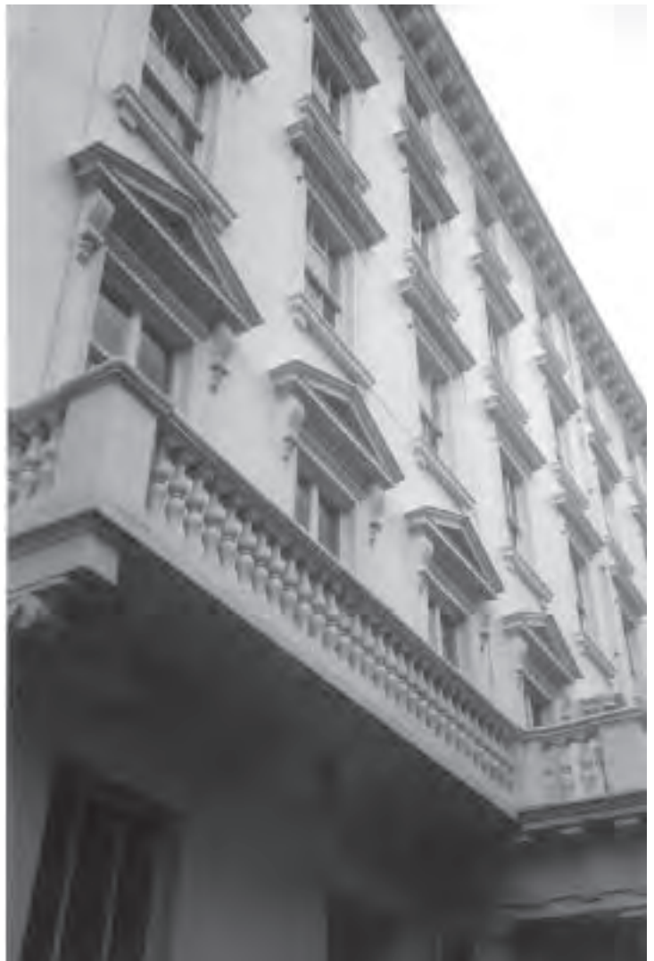
Stucco detailing to the entire facade
