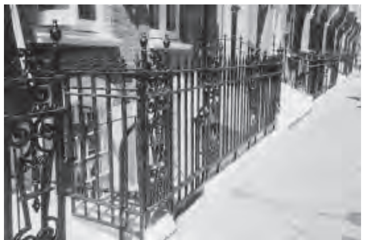
Cast iron railings
