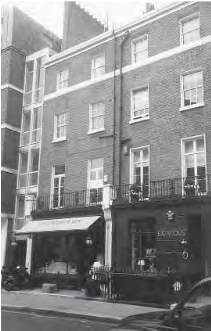
Nos. 4 and 6 Pont Street
