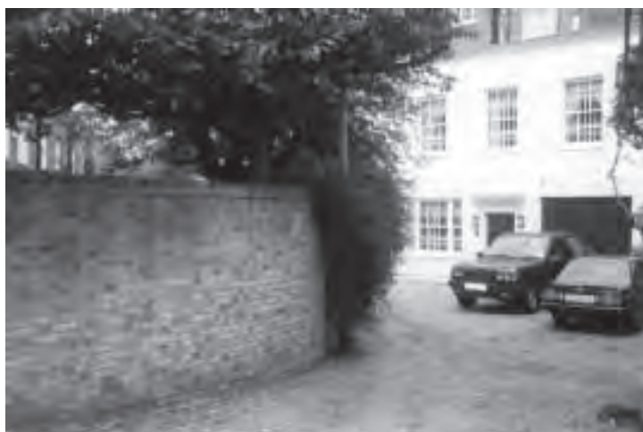
Curving wall above the course of the Westbourne River in West Eaton Place Mews
