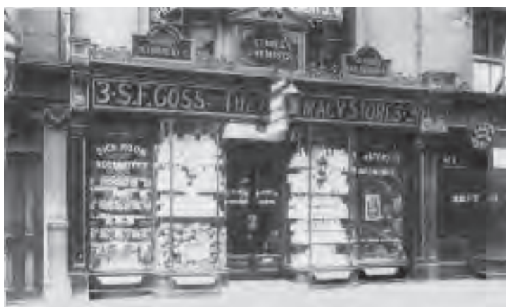
Turn of the century shopfront, Sloane Street ( now demolished )
