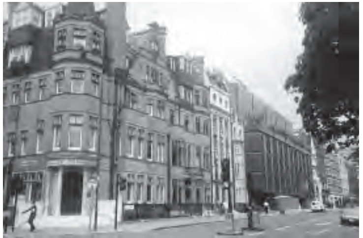
View north side of Sloane Street from Pont Street
