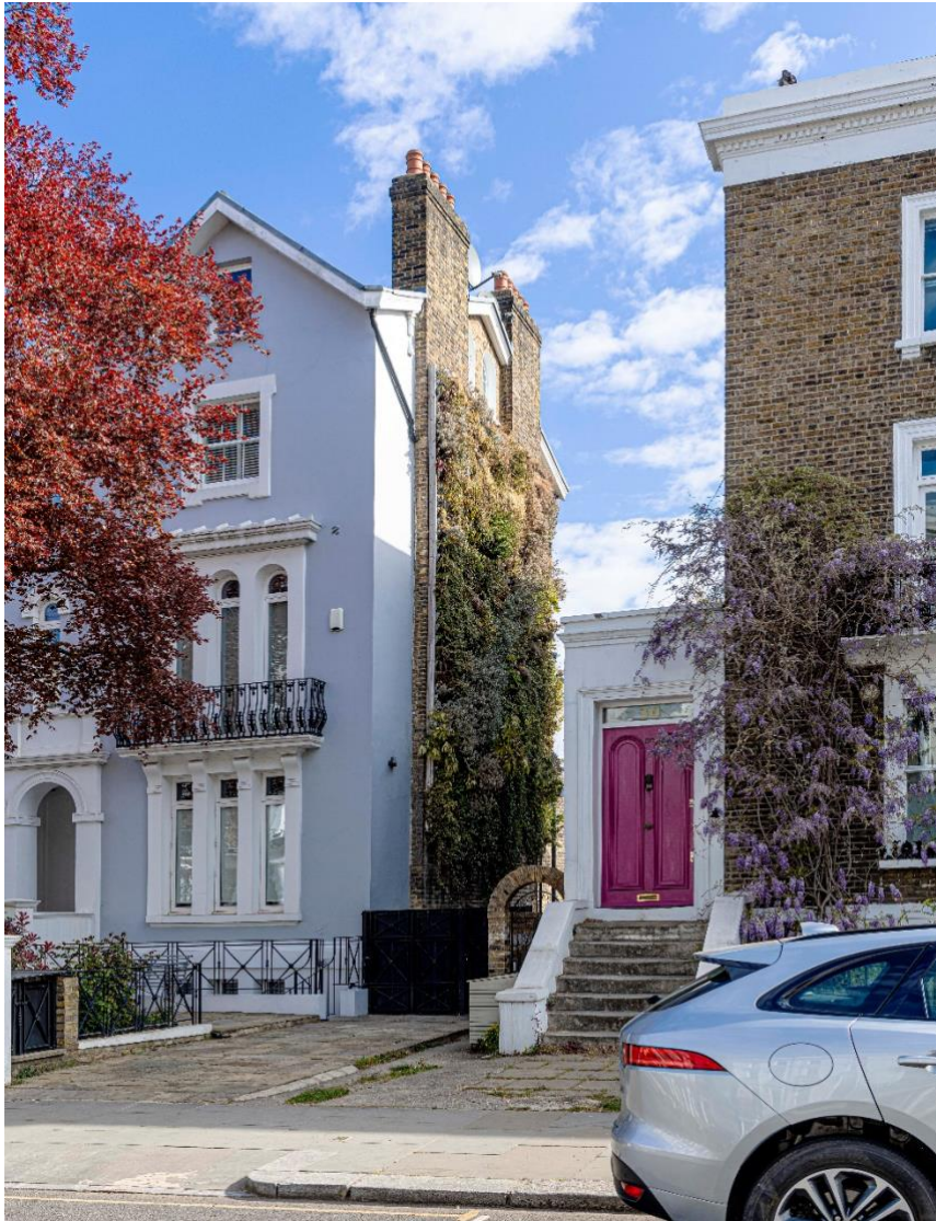
Figure 11.6: Green wall at 32 Kensington Park Road (photo credit: photoBECKET)
