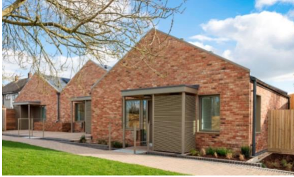
Suffolk Close, Bristol Low energy council housing designed by Emmett Russell architects using Passivhaus principles. Photograph: Craig Auckland/Fotohaus
