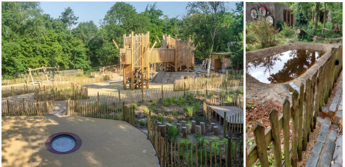
Figure 12.3: Example of SuDS in Holland Park (shallow attenuation basin above and award-winning adventure playground which incorporates SuDS)
