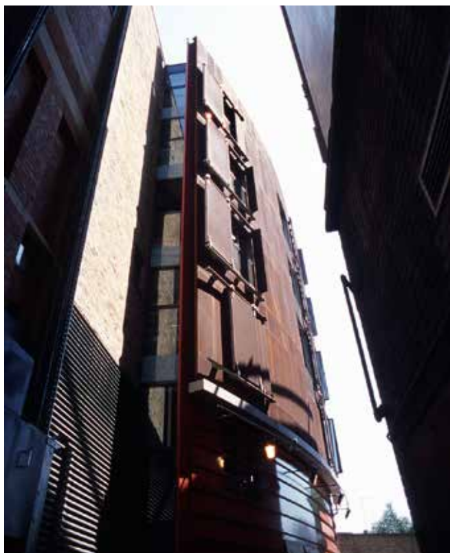
Extension to the Royal Court Theatre
