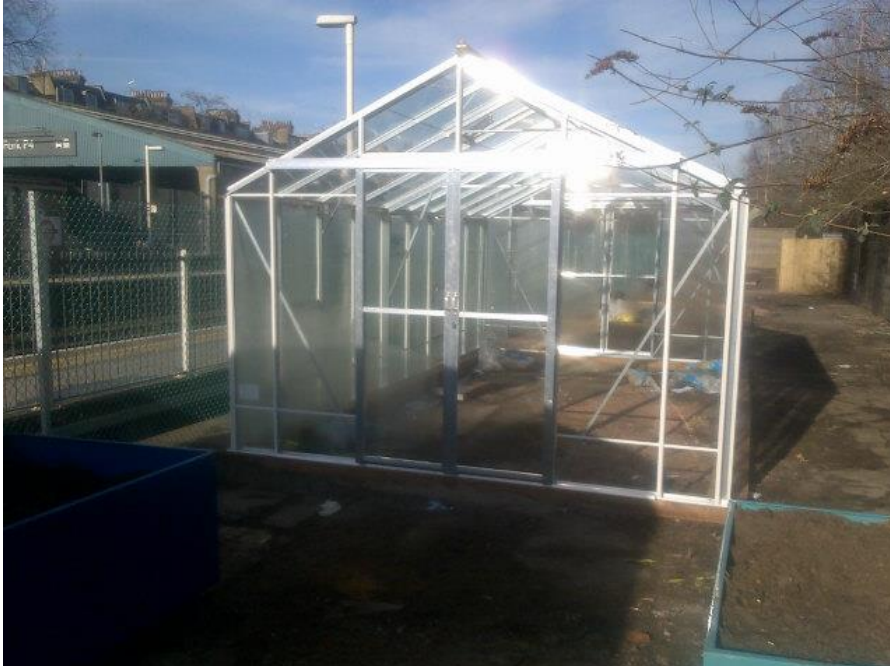
One of the new green houses being installed
