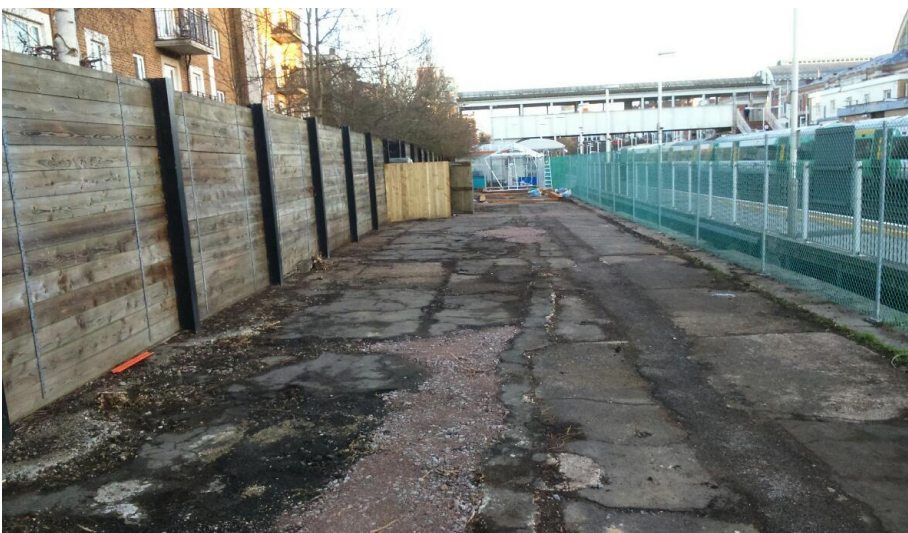
The cleared platform, ready for the new greenhouses
