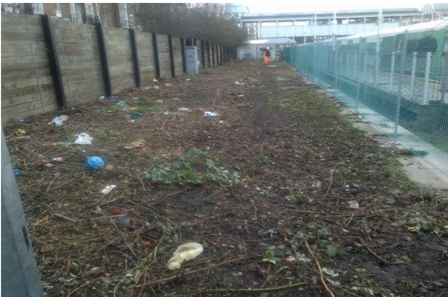
The platform being cleared and the new security fencing installed
