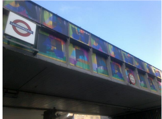
The repaired panels
