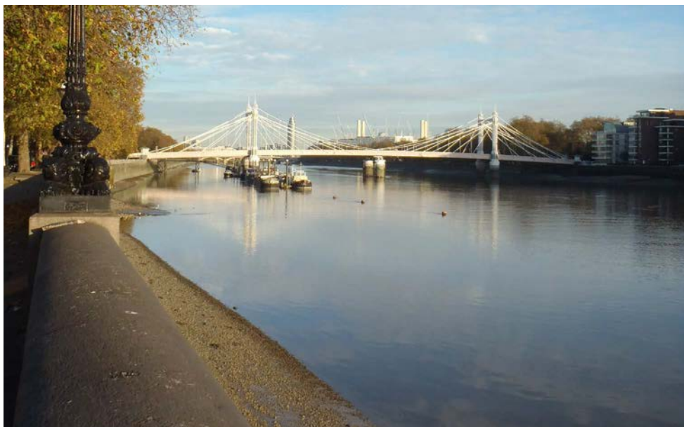
View of Albert Bridge from Chelsea Embankment
