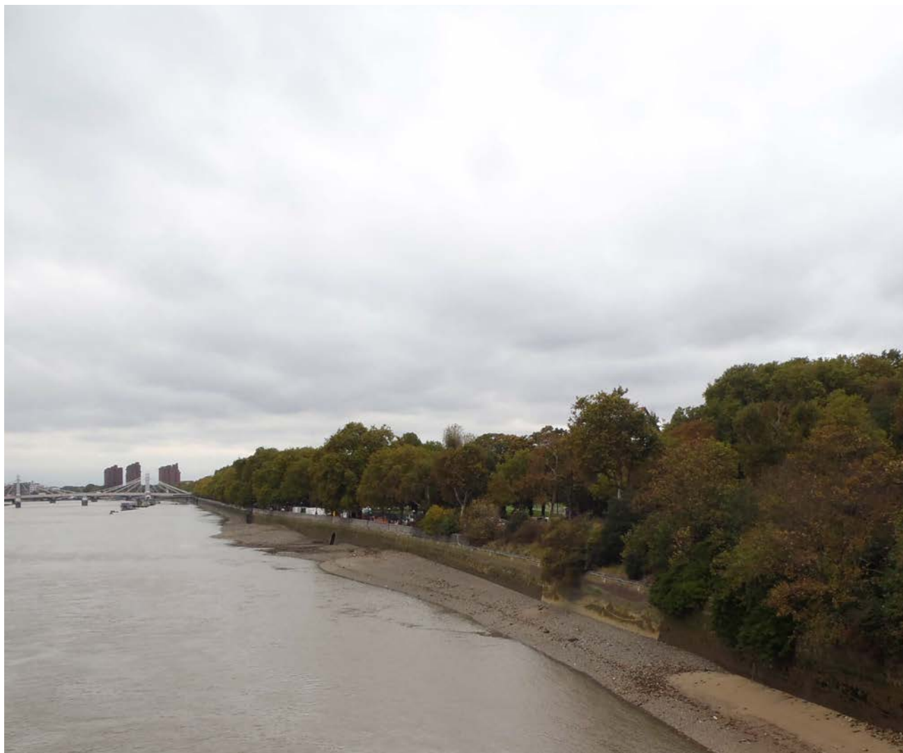
Chelsea Embankment river wall, grade II listed
