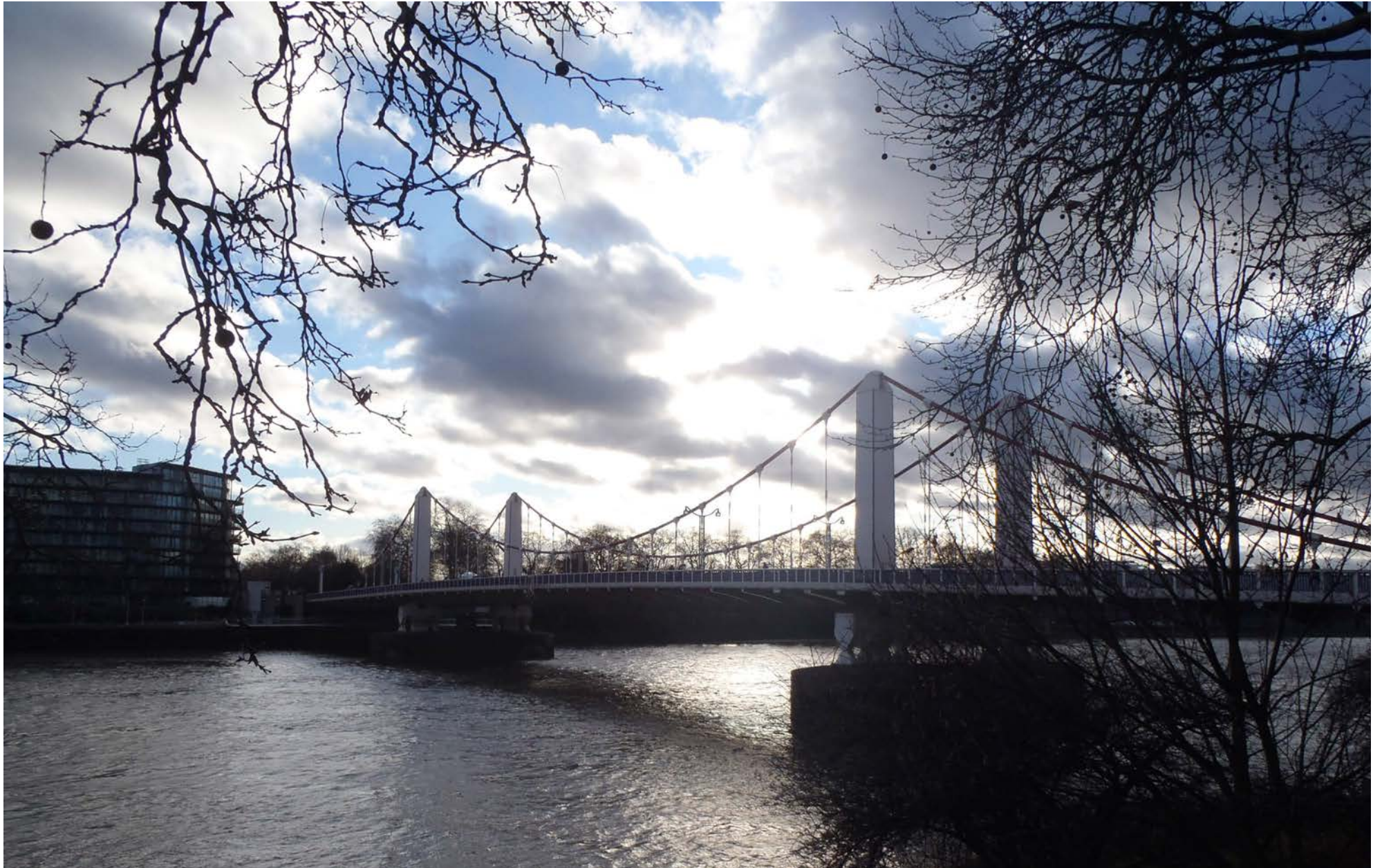
View of Chelsea Bridge from Grosvenor Road (outside of conservation area)
