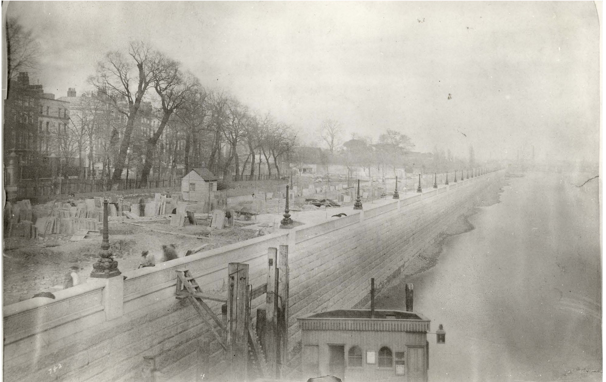
Chelsea Embankment under construction, photo by James Hedderly
