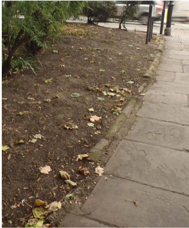
Missing original coping stones
