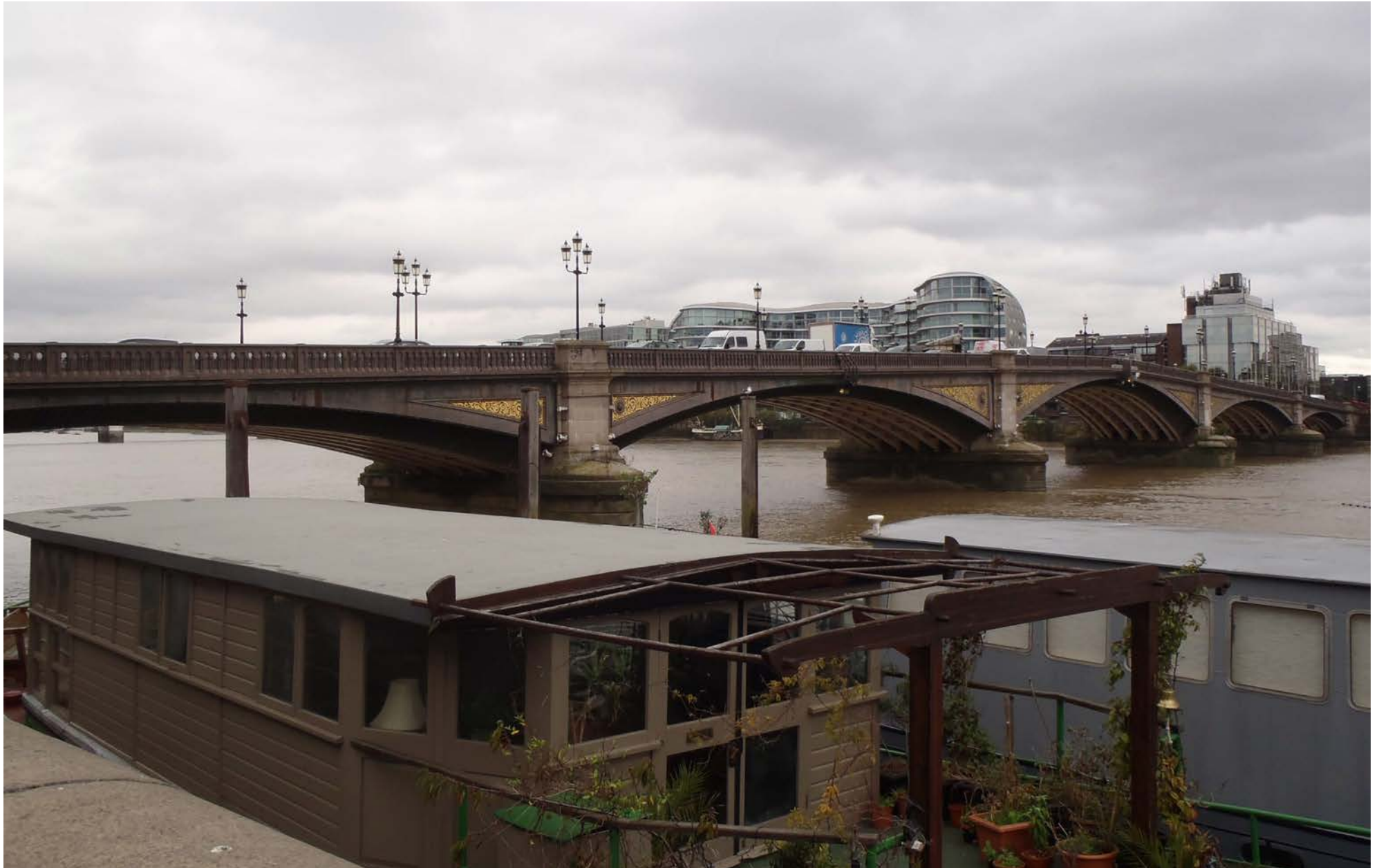
View of Battersea Bridge from Cheyne Walk
