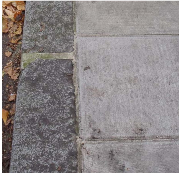
Granite kerbs and concrete slab paving
