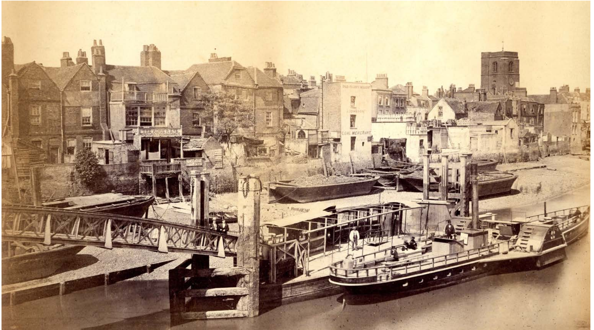
Old Ferry Wharf, photo by James Hedderly
