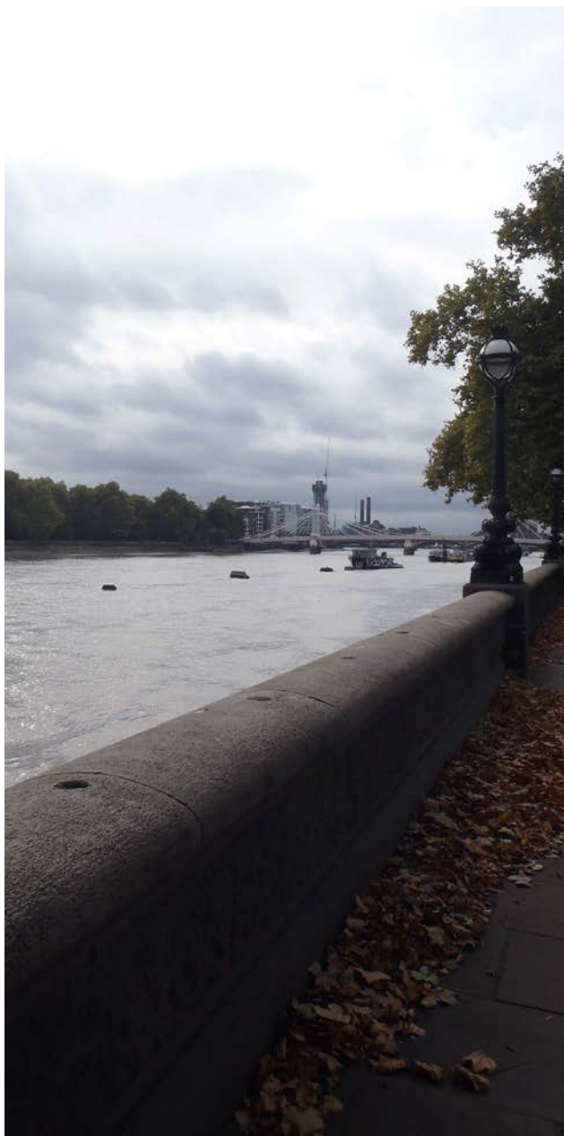
Hammer dressed granite wall, Chelsea Embankment
