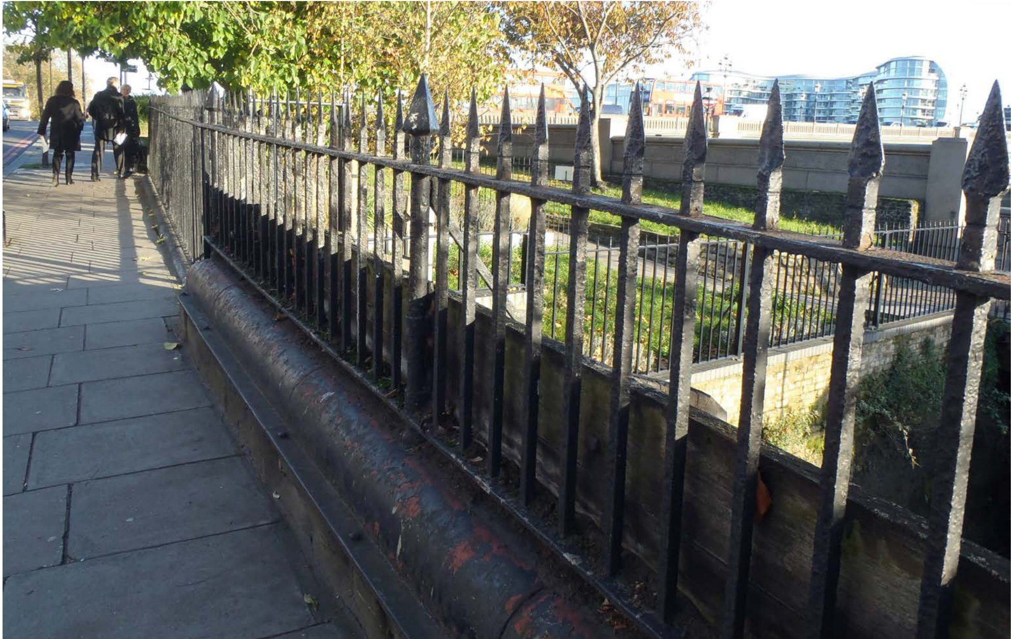
Metal railings, Battersea Bridge Gardens
