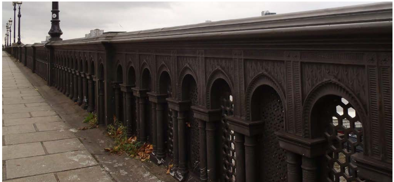
Pedestrian walkway on Battersea Bridge
