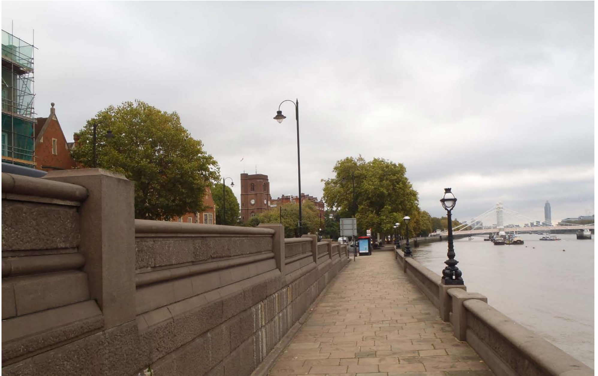
Chelsea Embankment, between Albert and Battersea Bridges
