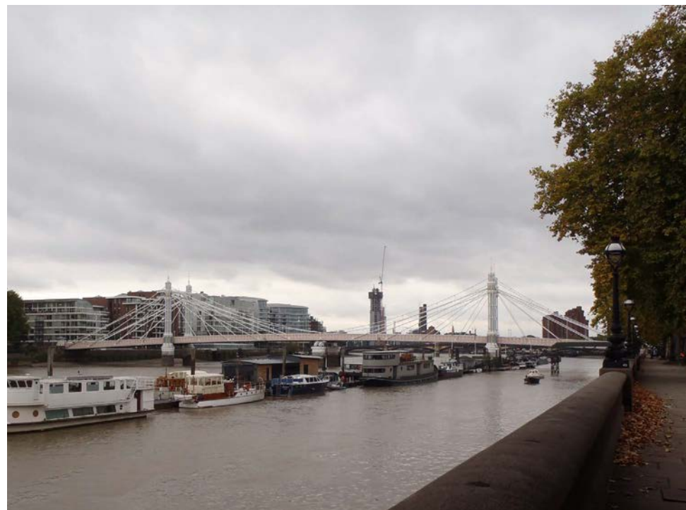
View of Albert Bridge from Chelsea Embankment
