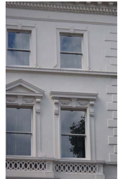
Timber window, glass and stucco
