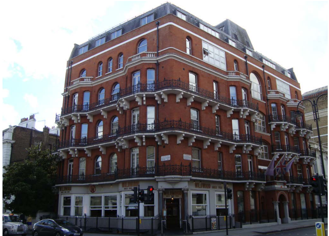
Nos. 154-156 (even) Gloucester Road
