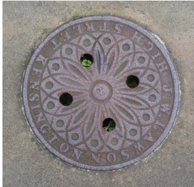
Cast iron coal hole covers
