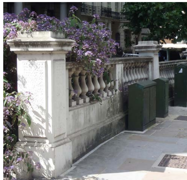
Bottle balustrades, Hyde Park Gate
