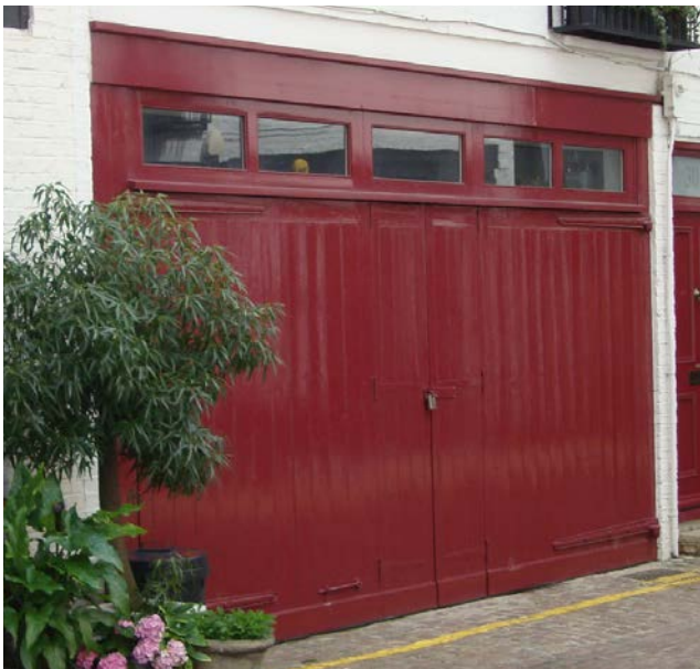
Closeboarded timber doors in a mews with toplights
