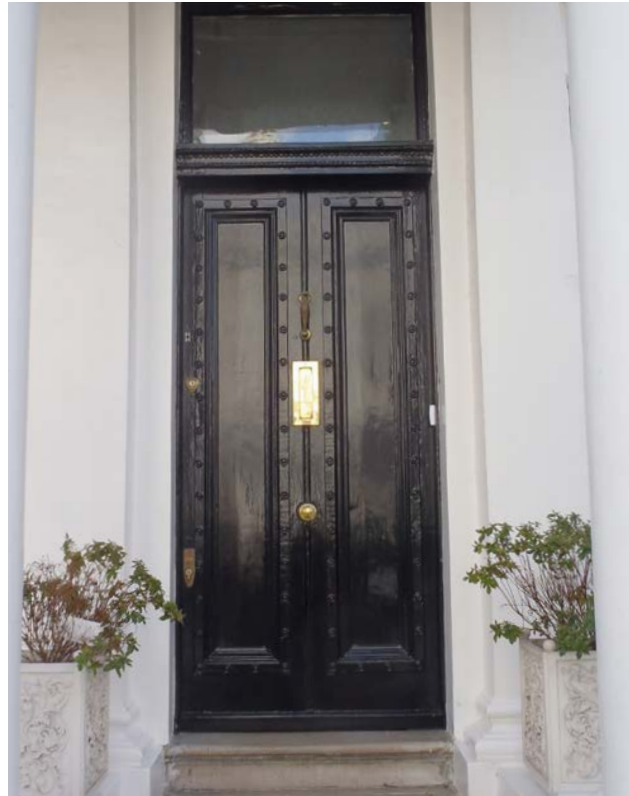
Two-panelled door, Kensington Gate
