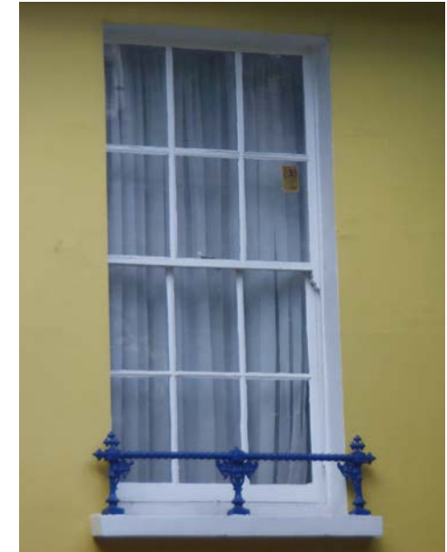
Six-over-six sash windows
