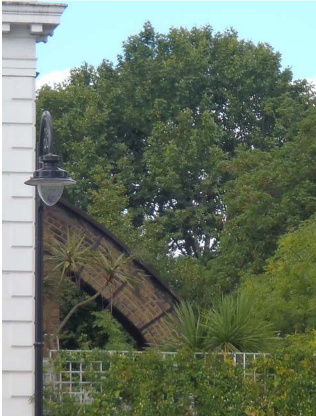
Arched chimney stack
