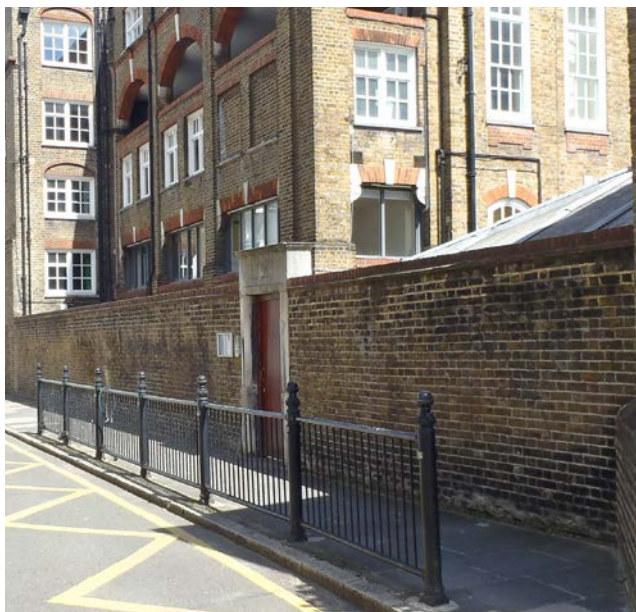
London Stock brick boundary wall
