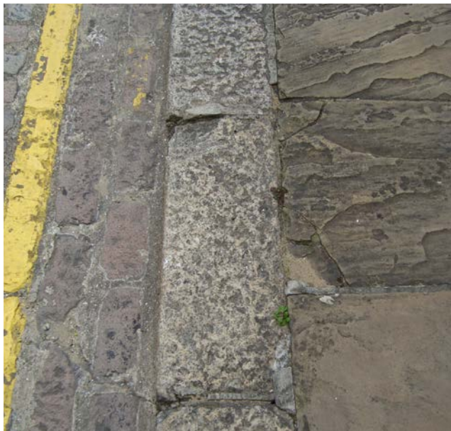
Granite kerbs, setts and York stone paving
