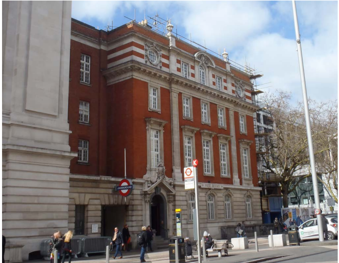
Former Post Office, no. 25 Exhibition Road and Pedestrian Subway
