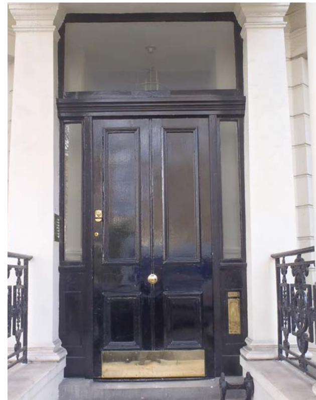
4-panelled door, Stanhope Gardens
