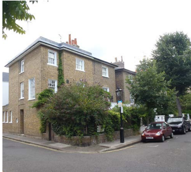
Gap between linked pairs of semi-detached houses, nos. 26 & 28 Clareville Grove
