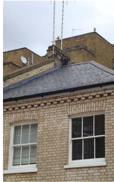
Natural slate roof
