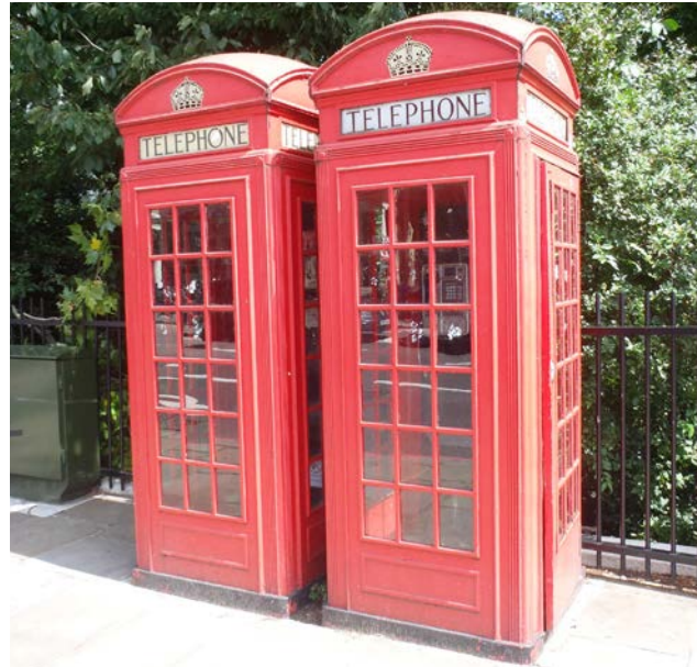
K6 cast iron telephone kiosks
