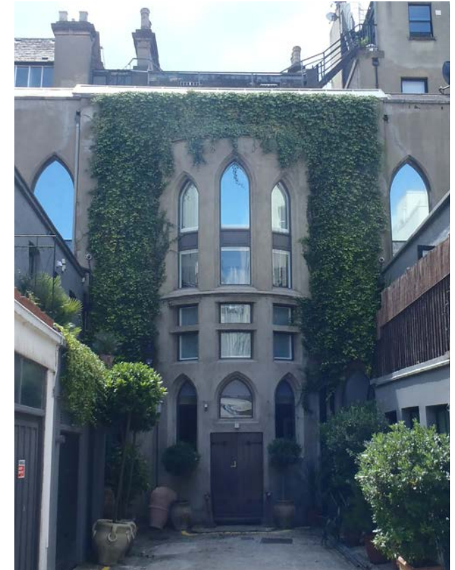
Rear of the former Queen's Gate Hall, nos. 40-42 (even) Harrington Road
