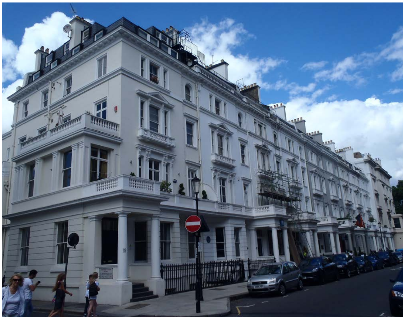
Nos. 2-18 (even) Queensberry Place
