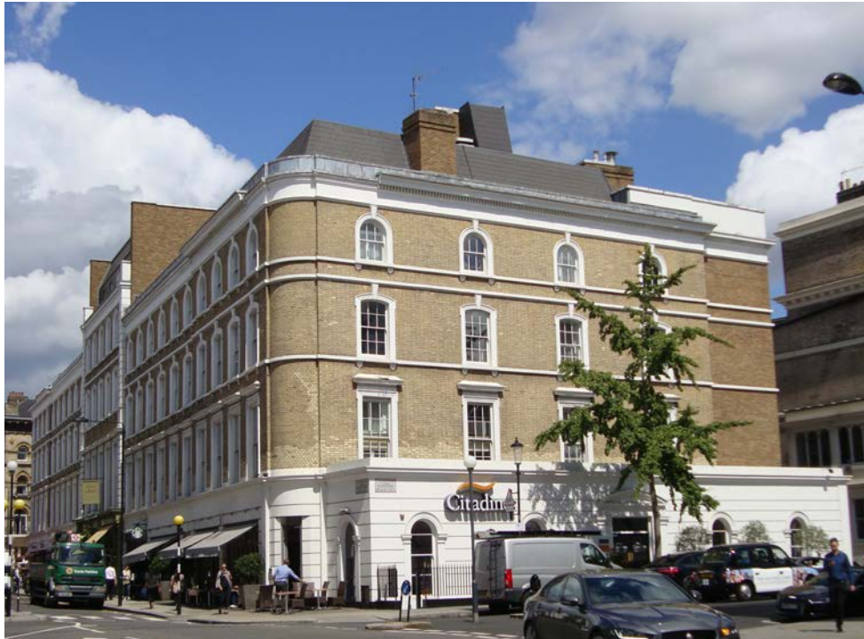
Nos. 17-35 (odd) Gloucester Road
