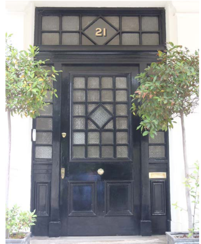
Elaborate glazing bars at no. 21 Queen's Gate Gardens
