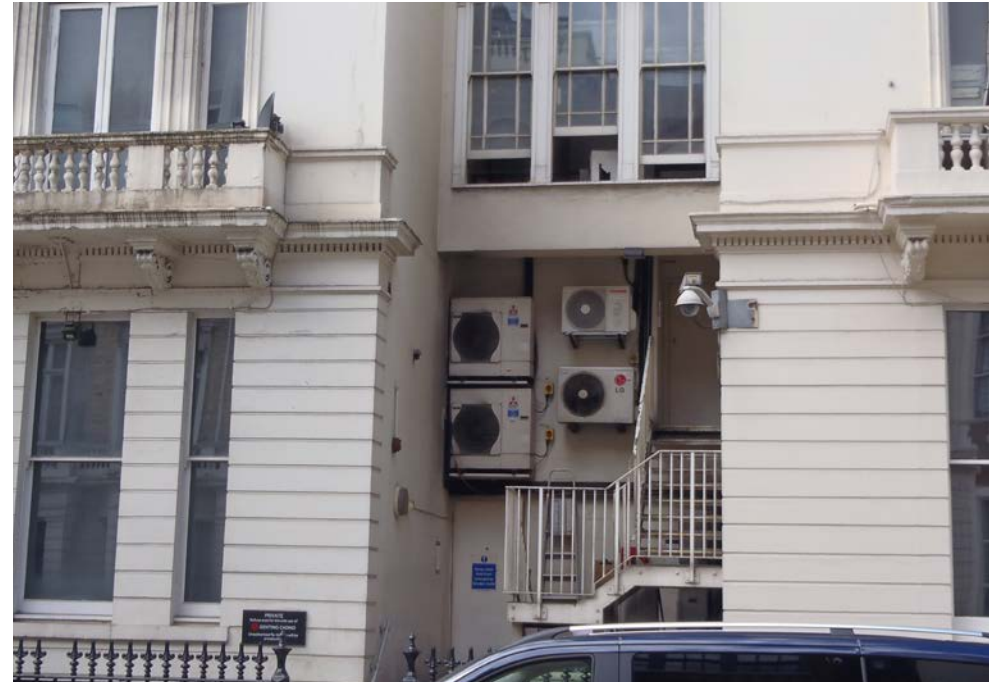
External clutter with air conditioning, staircase, satellite dish and security cameras
