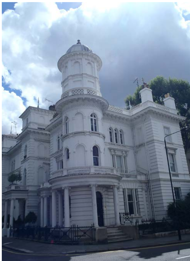
No. 1 Kensington Gate
