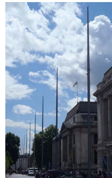
Contemporary mast lighting
