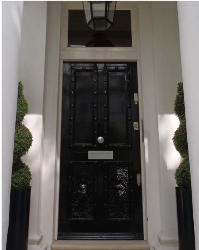
Decorative cast iron bottom panels, Kensington Gate
