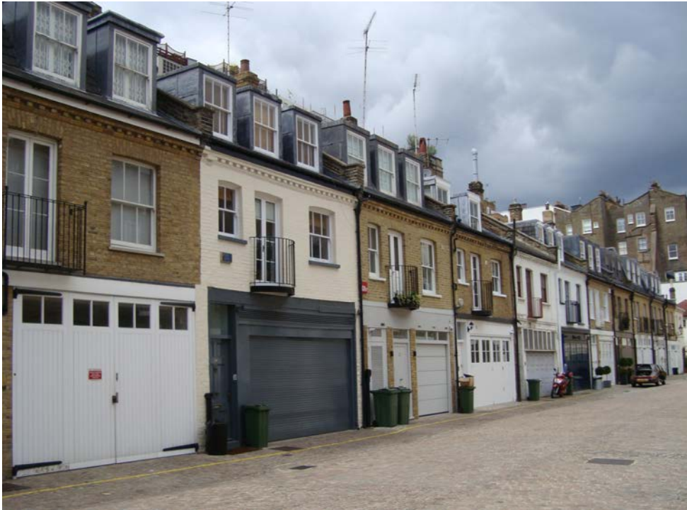
Western side of Queen's Gate Place Mews looking north
