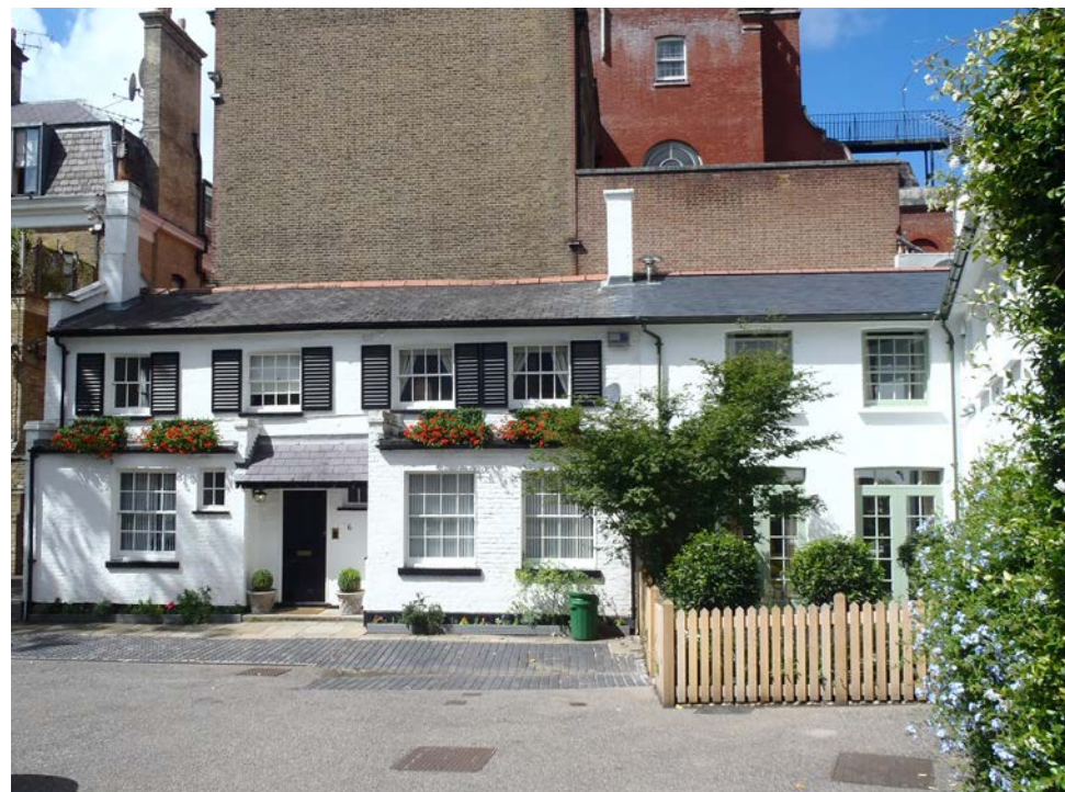
No. 6 and 7 Reston Place
