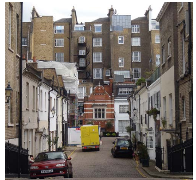
Elvaston Mews looking east on to no. 17
