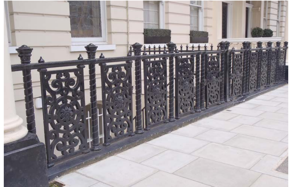
Railings to the south side of Queen's Gate Terrace
