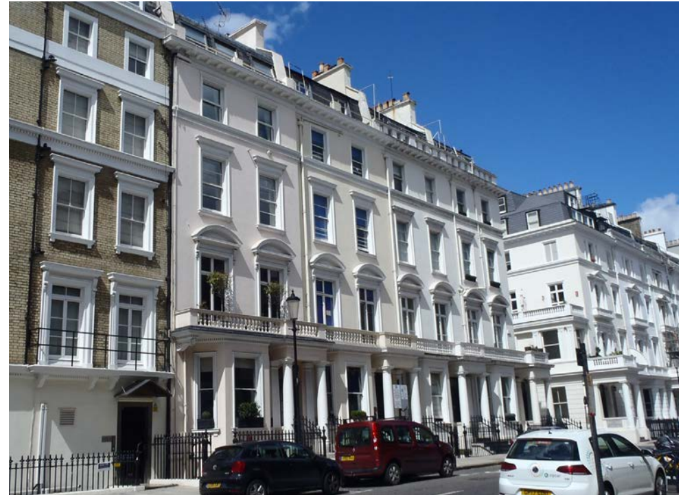
Nos. 20-26 (even) Queensberry Place
