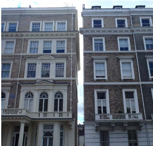
Gap between terraced groups, nos. 21 & 24 Queen's Gate Place
