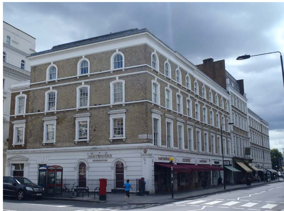
Nos. 17-35 (odd) Gloucester Road
