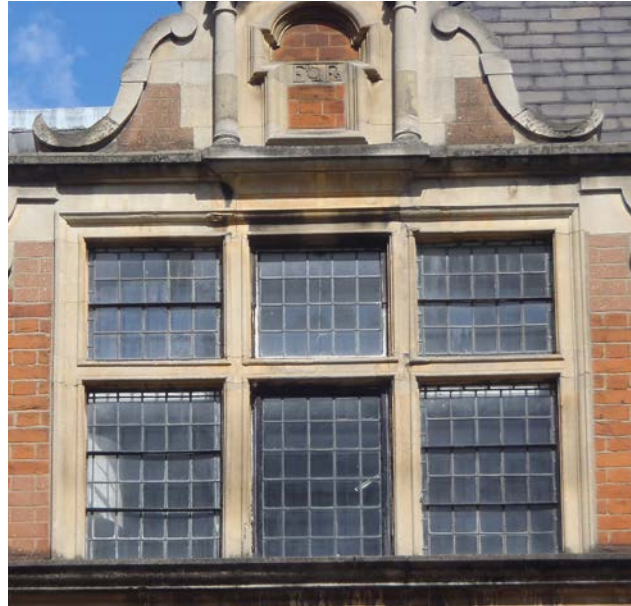
Mullion & transformed stone window
