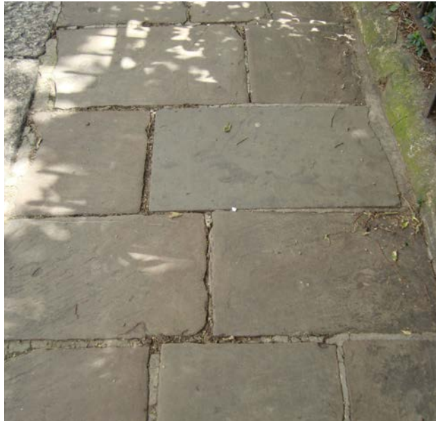
Riven York stone slabs, Hyde Park Gate
