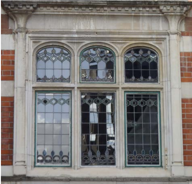
Mullion and transformed stone window with leaded casements
