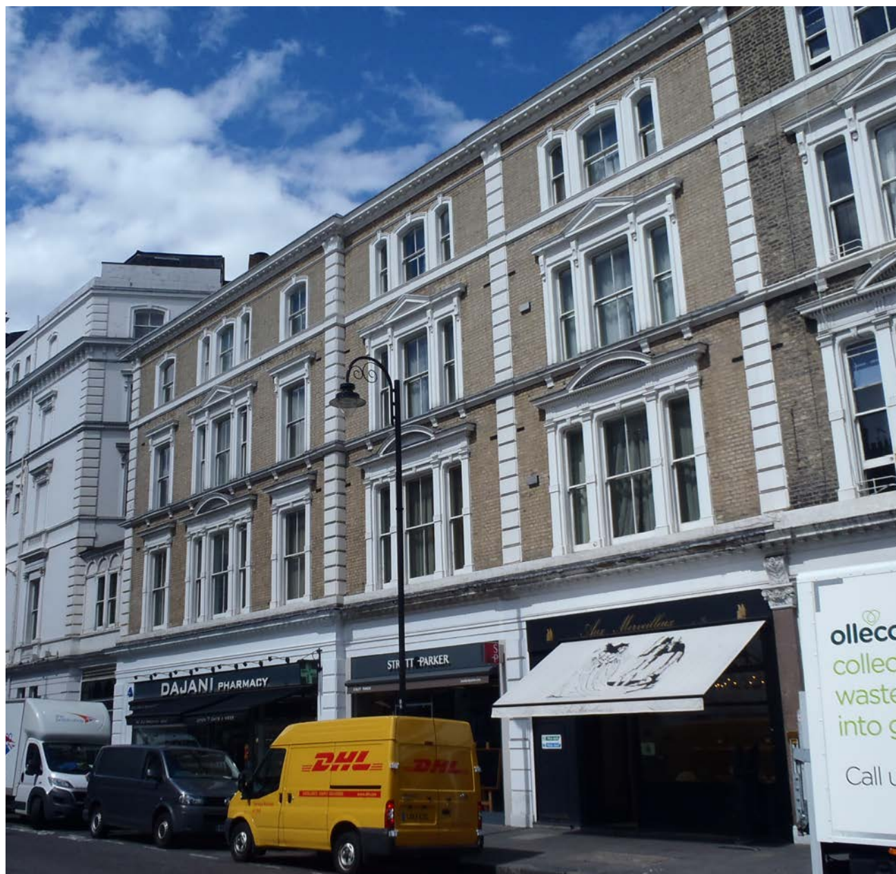
Nos. 88-92 (even) Old Brompton Road
