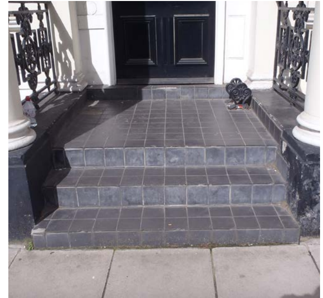
Tiled recladding of front entrance steps
