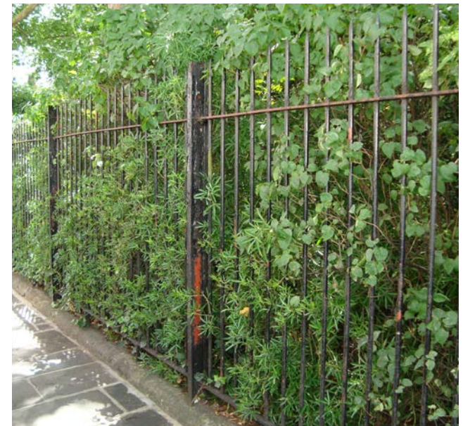
Non-original railings and I-beam posts, Queen's Gate Gardens
