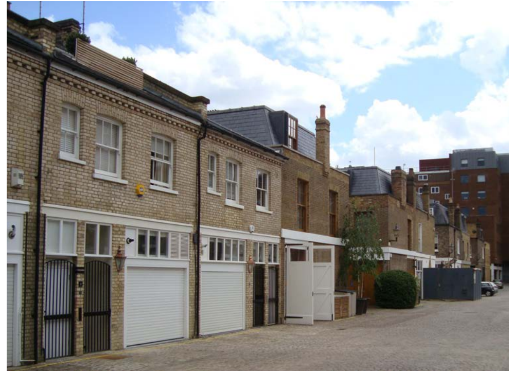
Eastern side of Queen's Gate Mews looking south
