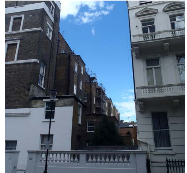
Gap between nos. 9-11 Queen's Gate revealing rear elevations
