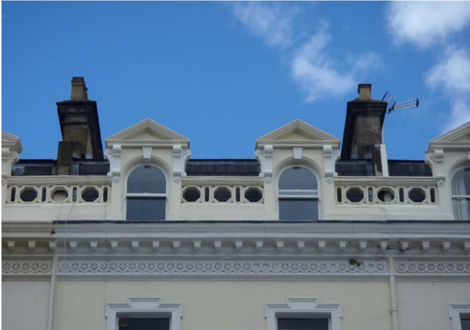
Mansard roof with masonry parapet
