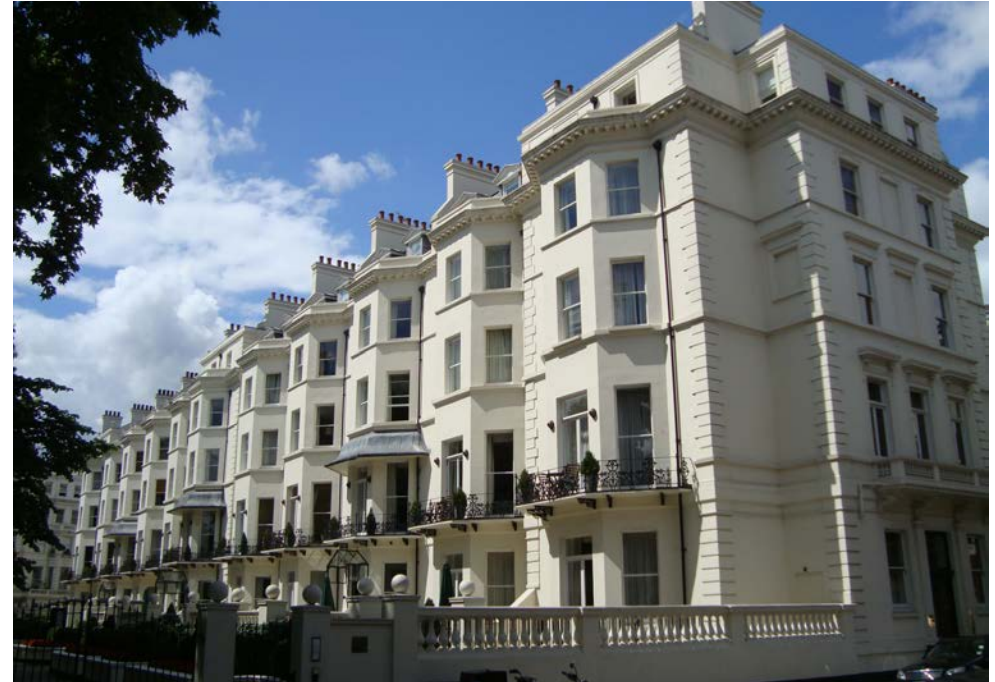
Formal stuccoed rear elevations to no. 75 Stanhope Gardens
