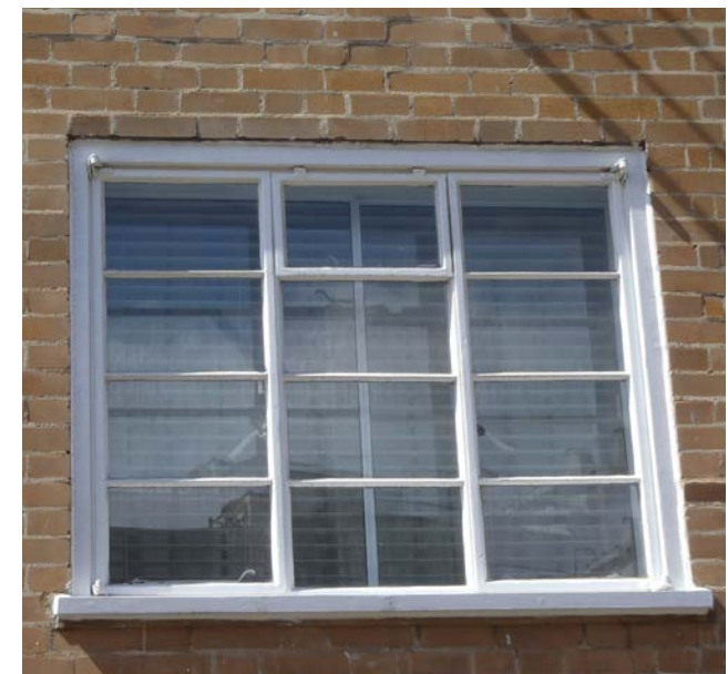
Metal casement window to a 1950s property
