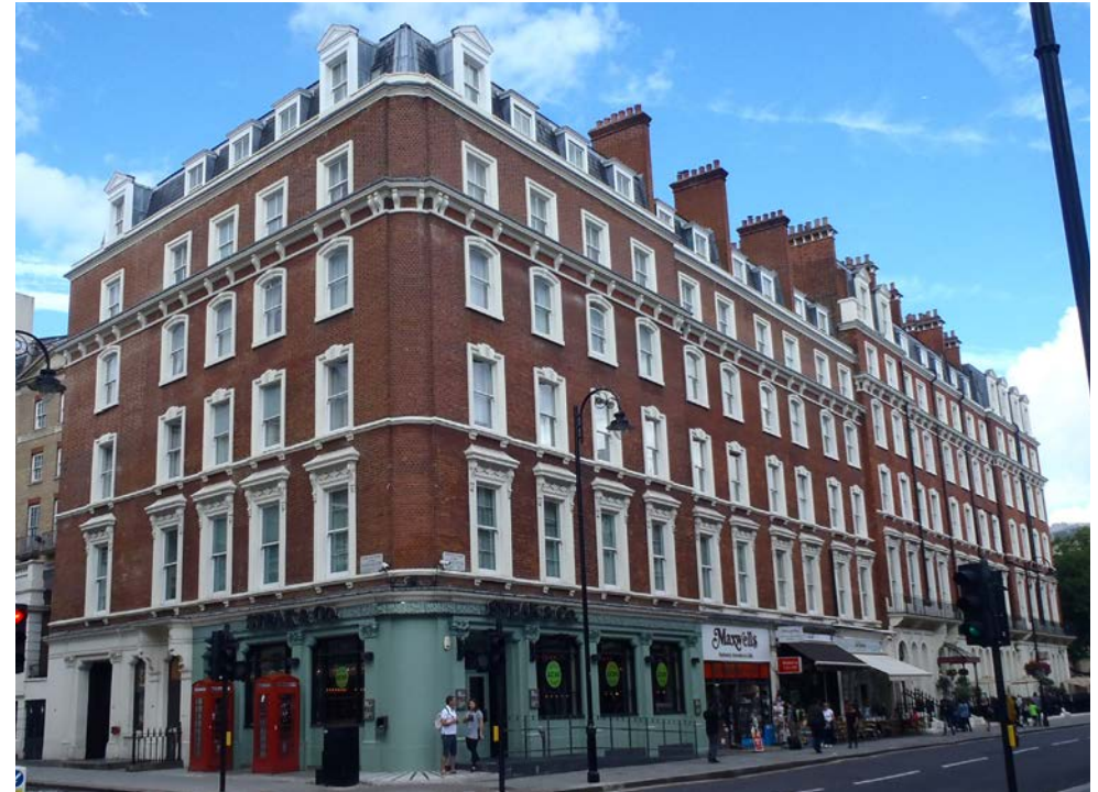
Nos. 144-152 (even) Gloucester Road
