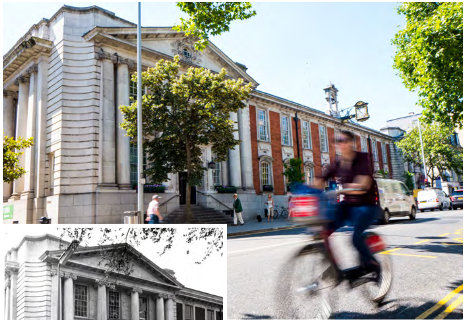
Chelsea Old Town Hall has been a London Landmark for generations. From bottom to top, you can see the Town Hall in the early 1900s, 1974 and 2018.
