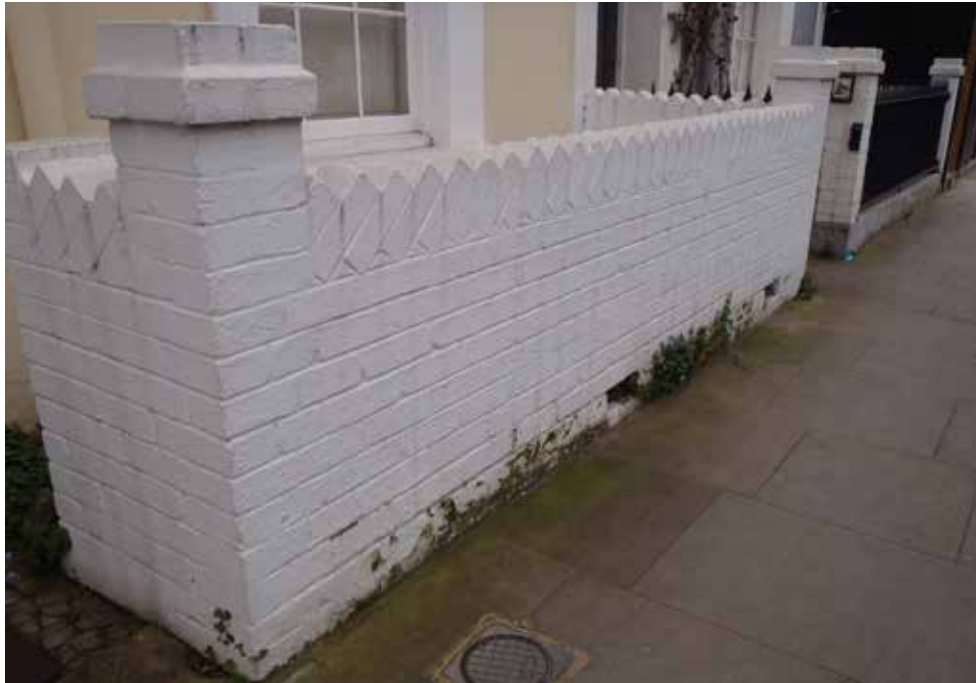
Modern replacement boundary wall in painted brick
