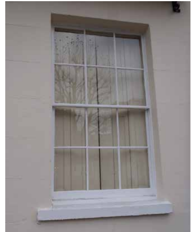
Six over six timber frame sash window
