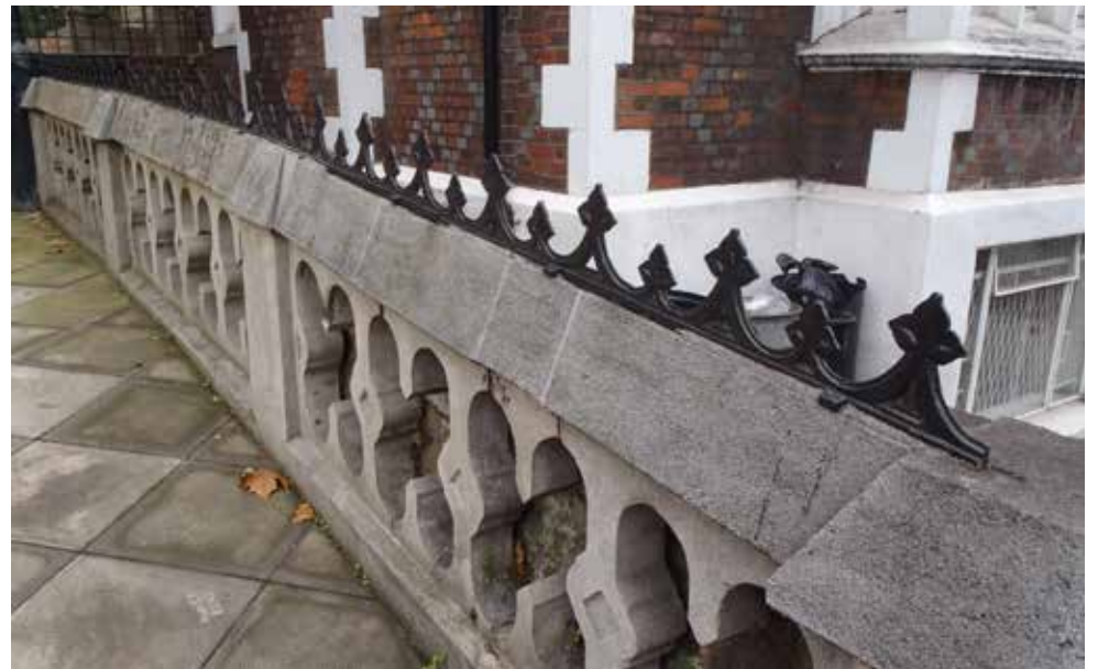
Pierced stone boundary wall, St. Ann's Villas
