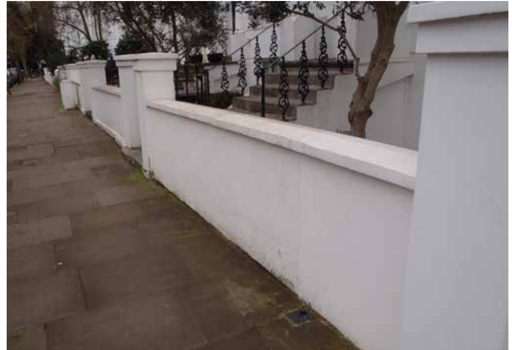
Stucco walls and gate piers
