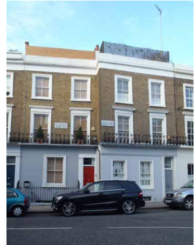
Trellising and timber balustrade on roofs
