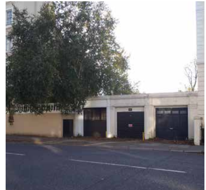
Garages, St Anns Villas
