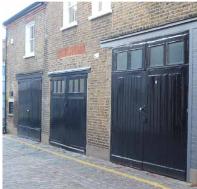
Mews garage doors, Addison Place
