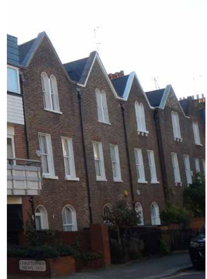
No. 22-28 (even) Penzance Street
