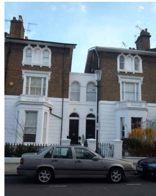
Nos. 32-34 (even) Portland Road
