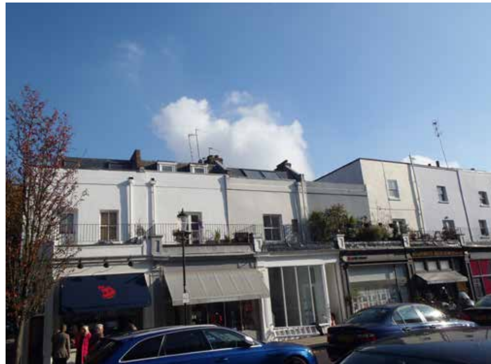
Nos 6-14 (even) Portland Road
