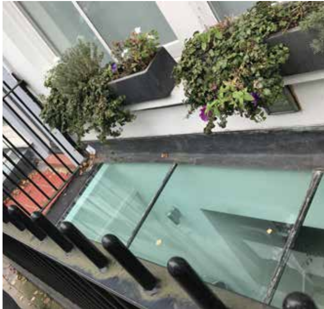
Lightwell blocked by glass
