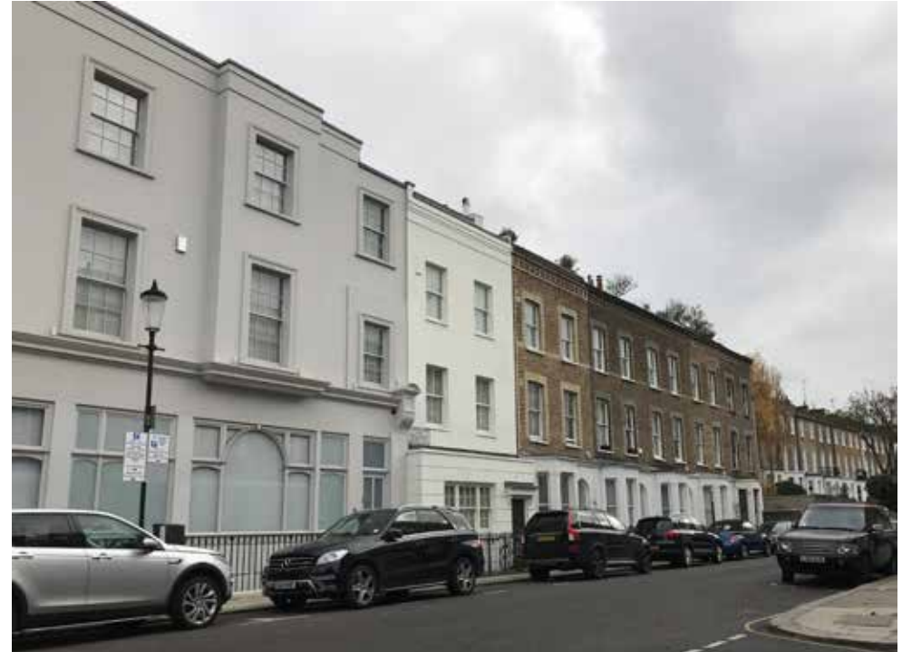
Nos. 2-14 (even) Princesdale Road
