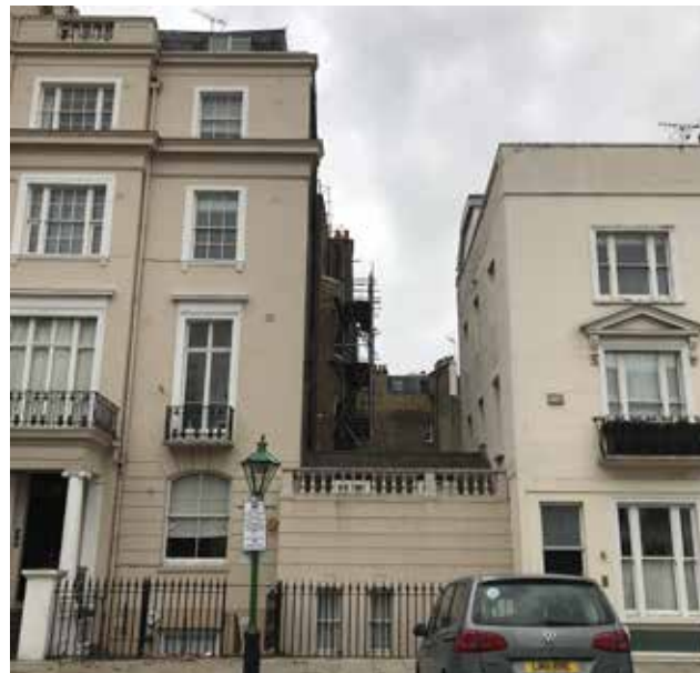
Rear of 170 Holland Park Avenue from Addison Avenue
