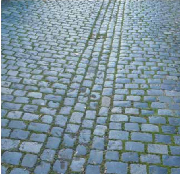
Granite setts and gully
