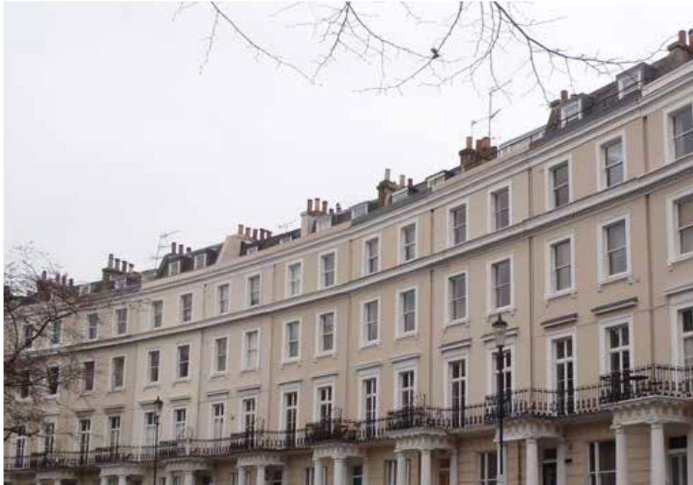
Front parapets and mansards, Royal Crescent
