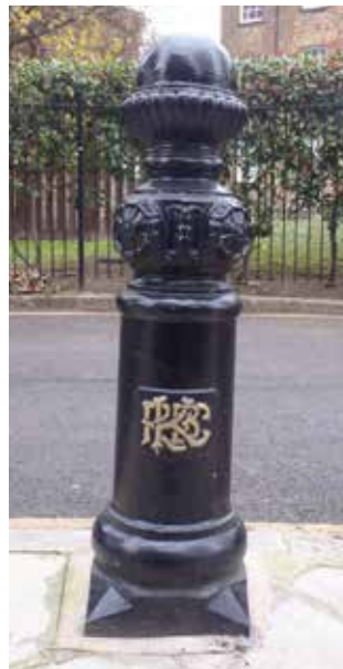
Cast iron bollards
