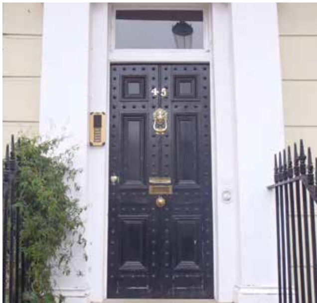
Six panelled door with studded nail decorations
