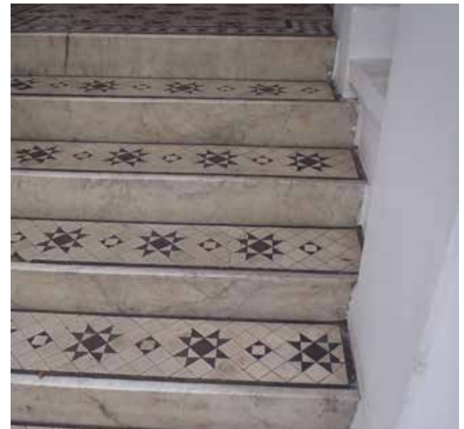
Tiled entrance steps
