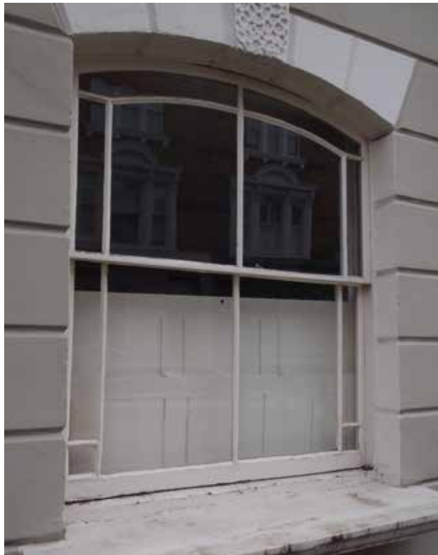
Two over two timber sash windows with margin lights
