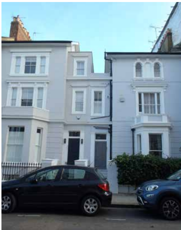
Nos. 56-58 (even) Portland Road
