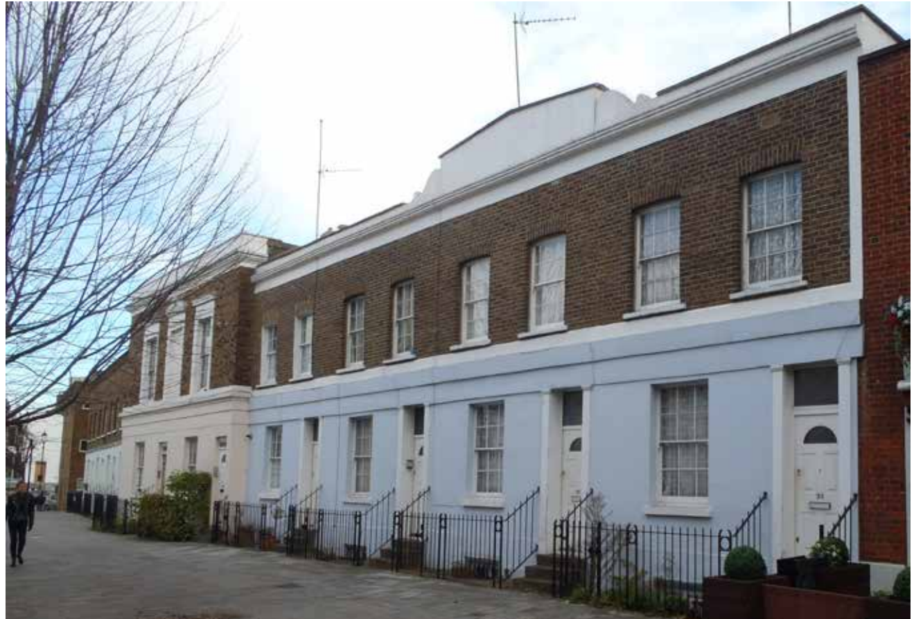
Nos. 30-50 (even) Norland Road
