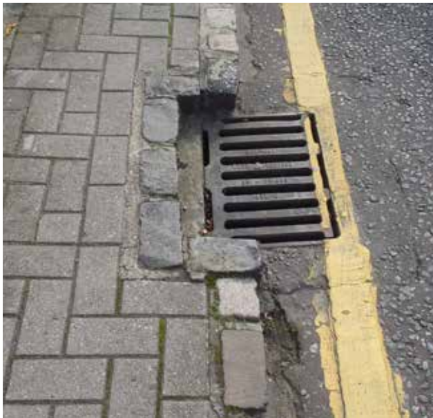
Concrete block paving
