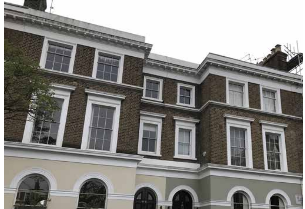
Parapets, St. James's Gardens
