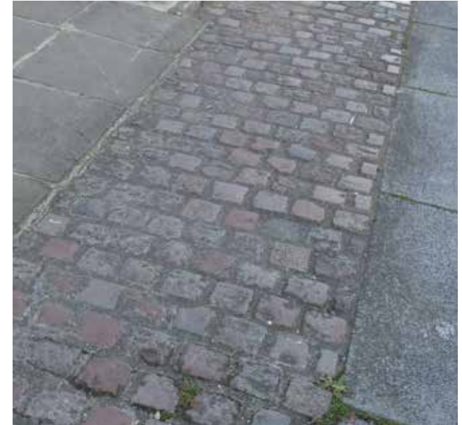
Granite kerbs, setts and York stone paving
