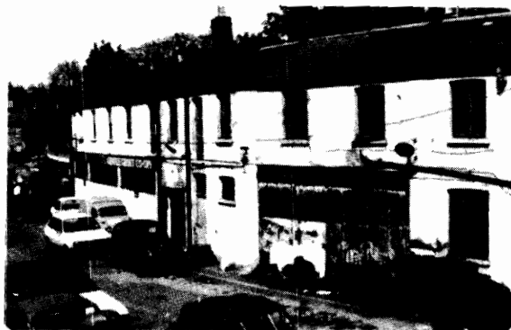
Royal Crescent Mews, south end cottages
