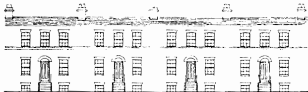
Princes Place now demolished
