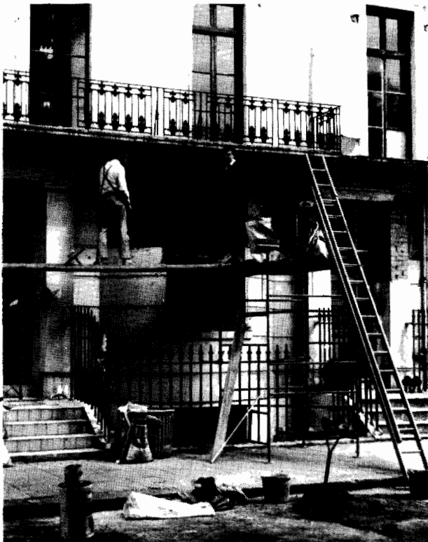
Restoration of stucco Norland Square
