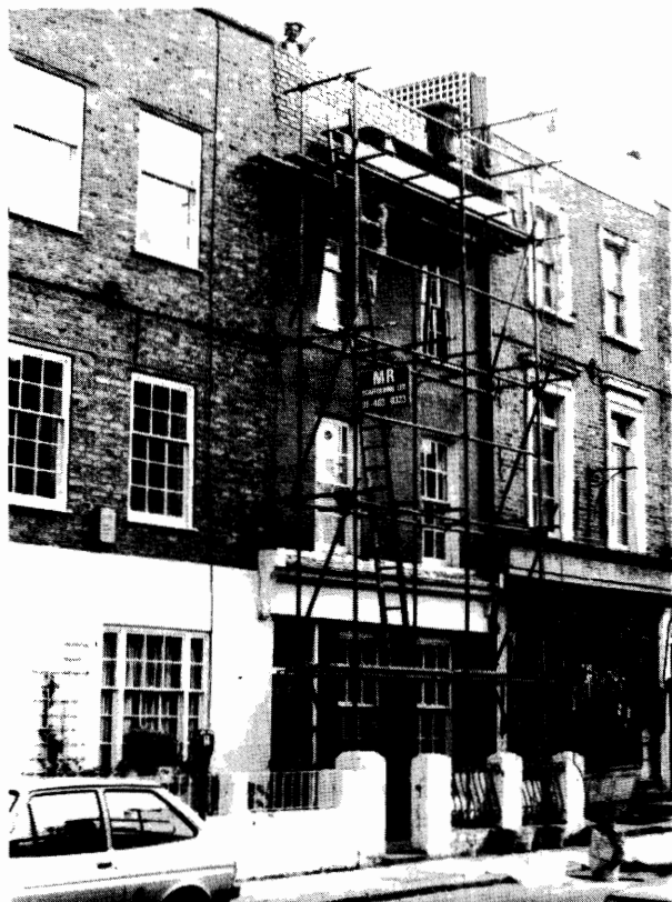
Restoration and repair Princedale Road.
