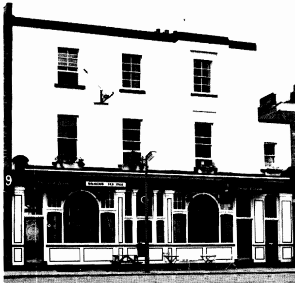
Missing cornices and glazing bars
