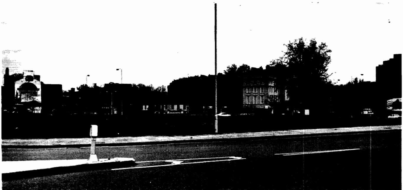
View towards the Norland Area across the Holland Park Avenue roundabout before landscaping.
