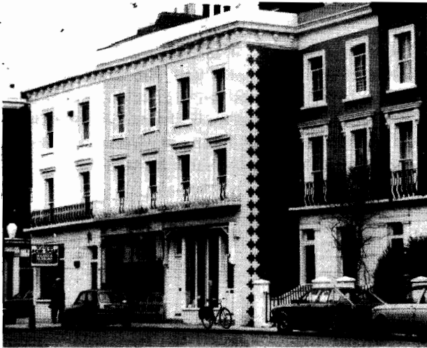
96, 98, 100 Portland Road: shop frontages.
