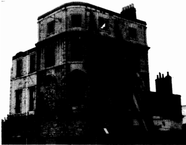
Norland Road before work started.
