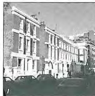
1 59-69 Palace Gardens Terrace
