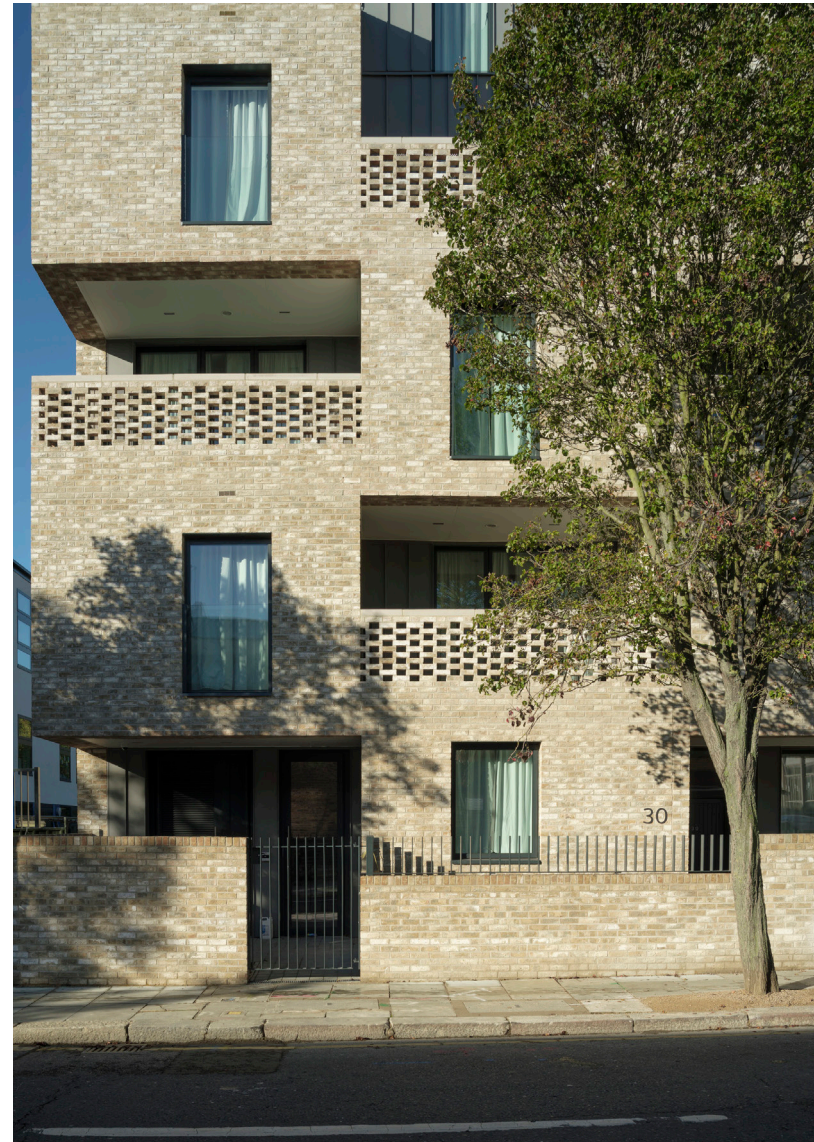
Middle Row Housing, by Penoyre & Prasad for RBKC © Greg Penoyre Housing Design Awards 2013, 'Projects Award' Winner
