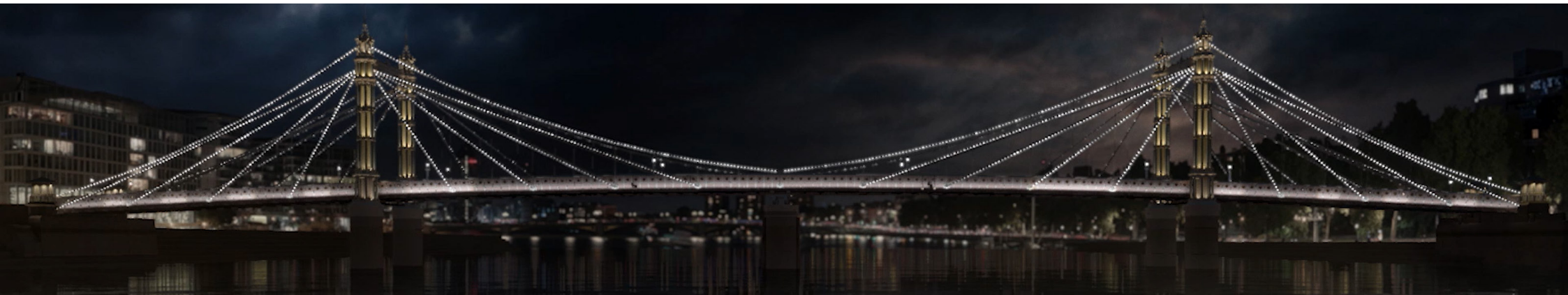
Albert Bridge, the Illuminated River project, conceived by artist Leo Villareal and Lifschutz Davidson Sandilands, delivered by a team including Icen Projects © Leo Villareal Studio
