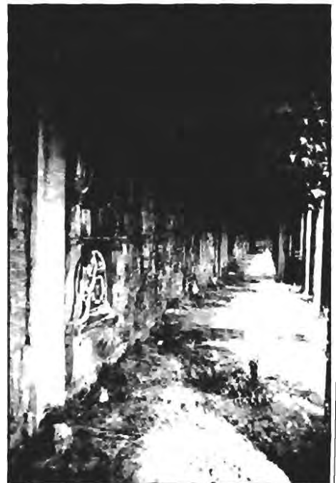
Damage to the Colonnade
