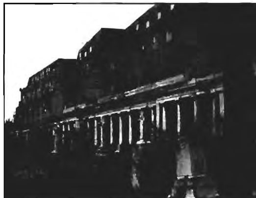
The hostel block - a damaging impact on the appearance of the colonnade
