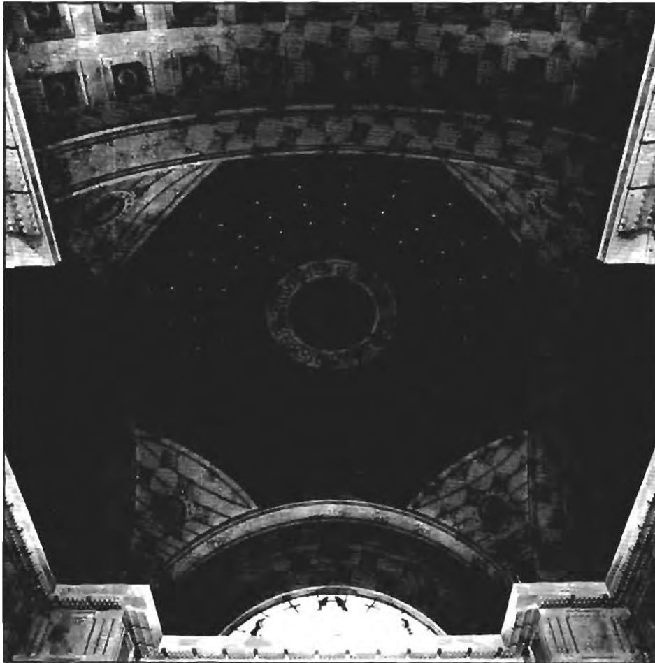
Ceiling of the Anglican Chapel
