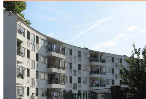
Kensal House Progressive, modernist estate designed for the working class who had previously lived in slums.
