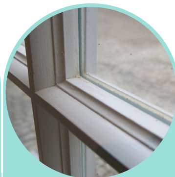
Thermally efficient glazing within existing frames
