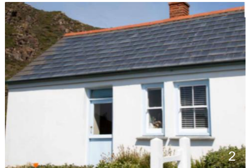
1 Solar PV on a flat roof integrated with a green roof, University of Greenwich 2 Example of integrated tiled PVs
