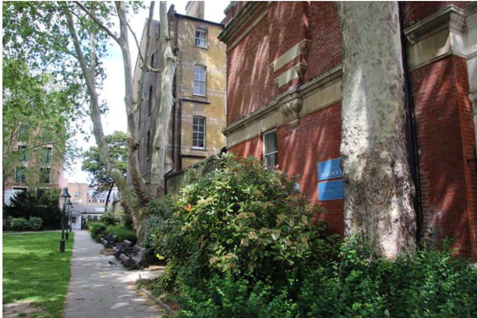
The western elevations of 151 Sydney Street and 250 King's Road are directly adjacent to Dovehouse Green. Special consideration should be given to this ancient burial ground when redeveloping these two buildings.
