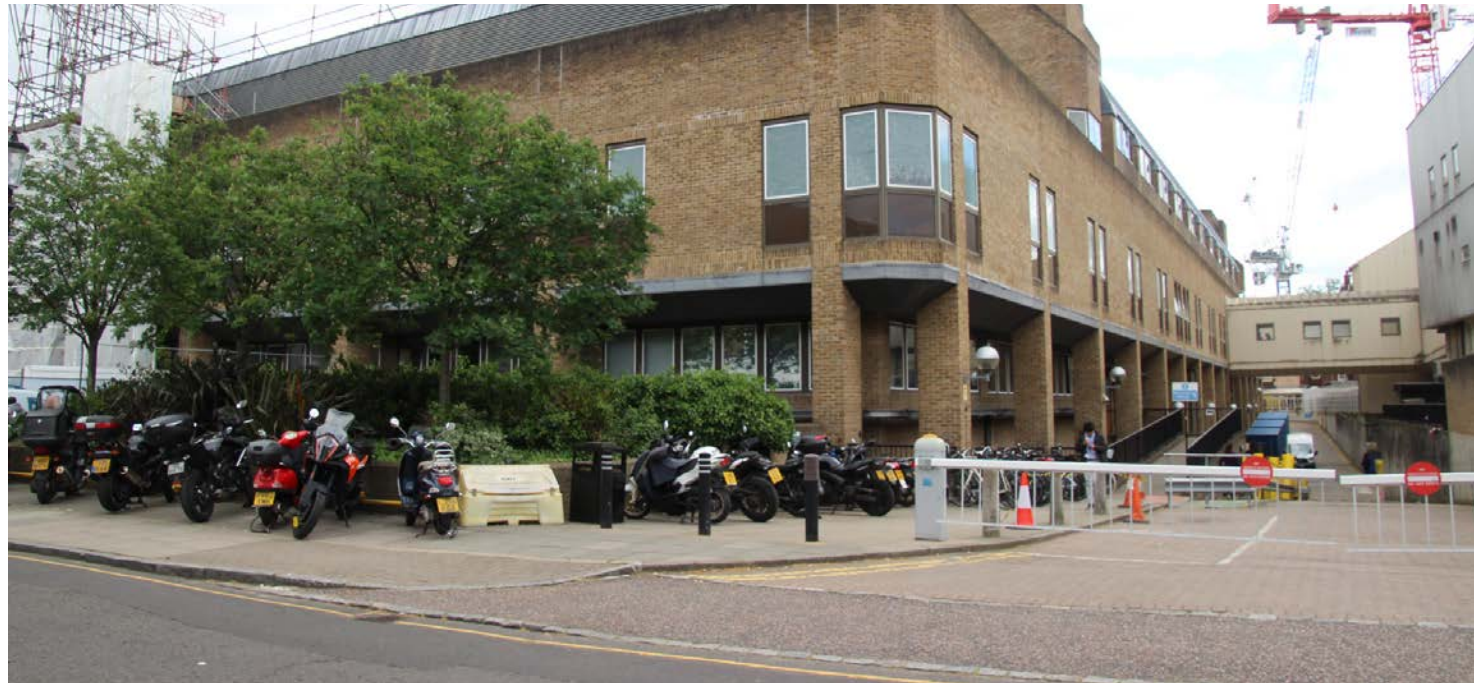
Public realm is generally of poor quality; it is currently dominated by hardscaping and vehicular parking with soft landscaping limited to occasional trees and shrubs.
