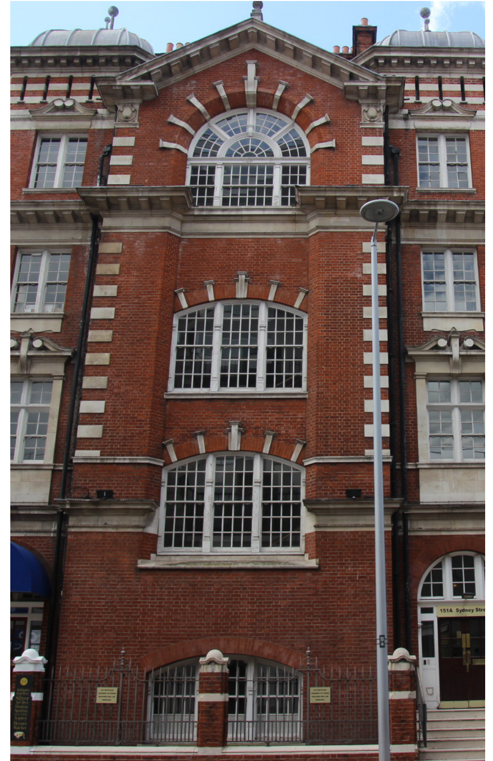
151 Sydney Street (east elevation). Red brick with stone detailing is a style of architectural detailing that is characteristic of the area.
