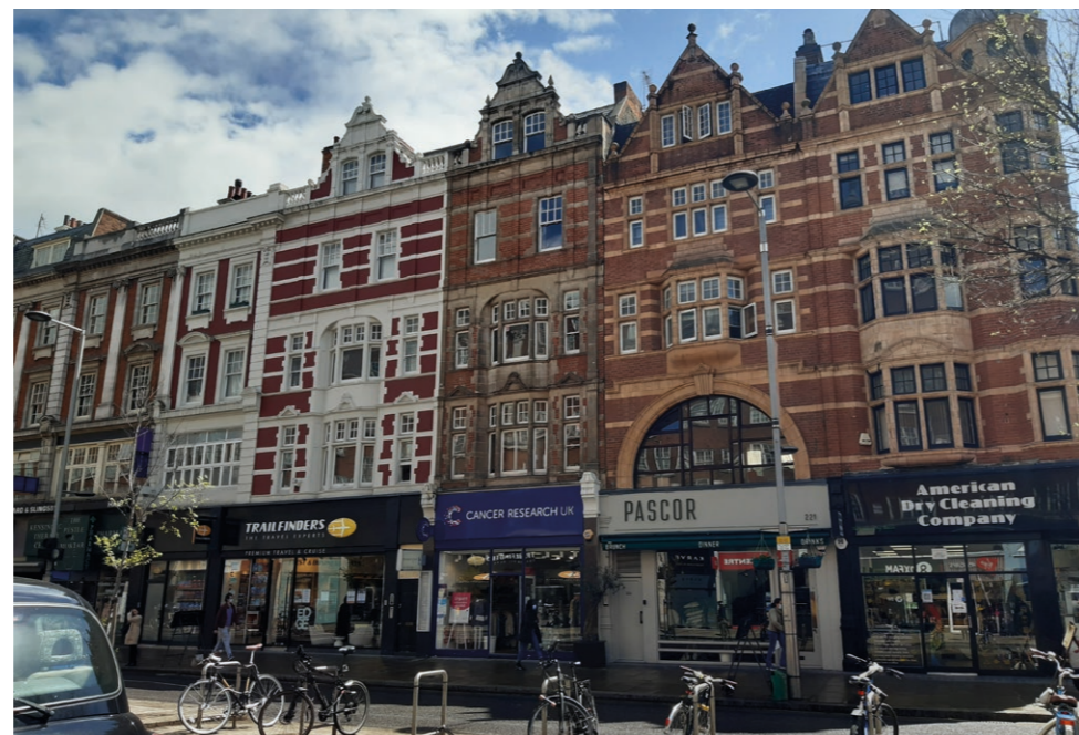
Varied roofline along Kensington High Street
