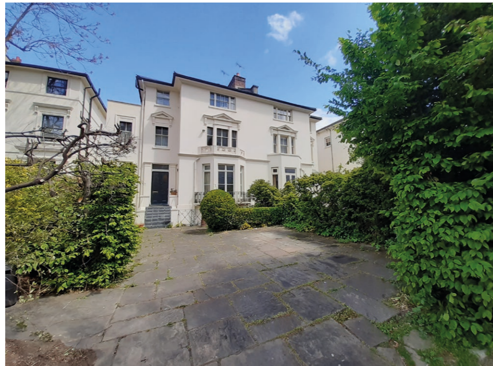
Gaps between buildings
