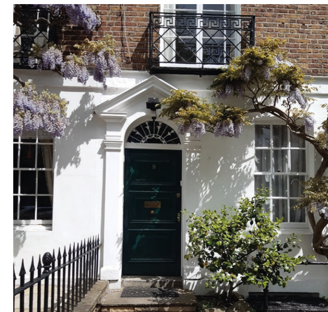
Decorative front entrance and balcony
