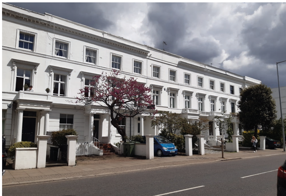
Consistent roofline behind a parapet
