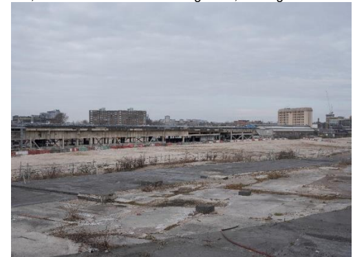
View to North-West with Ashfield House on Right in Background
