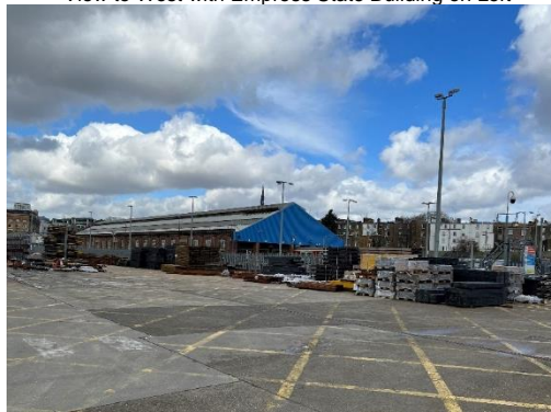
Lillie Bridge Depot
