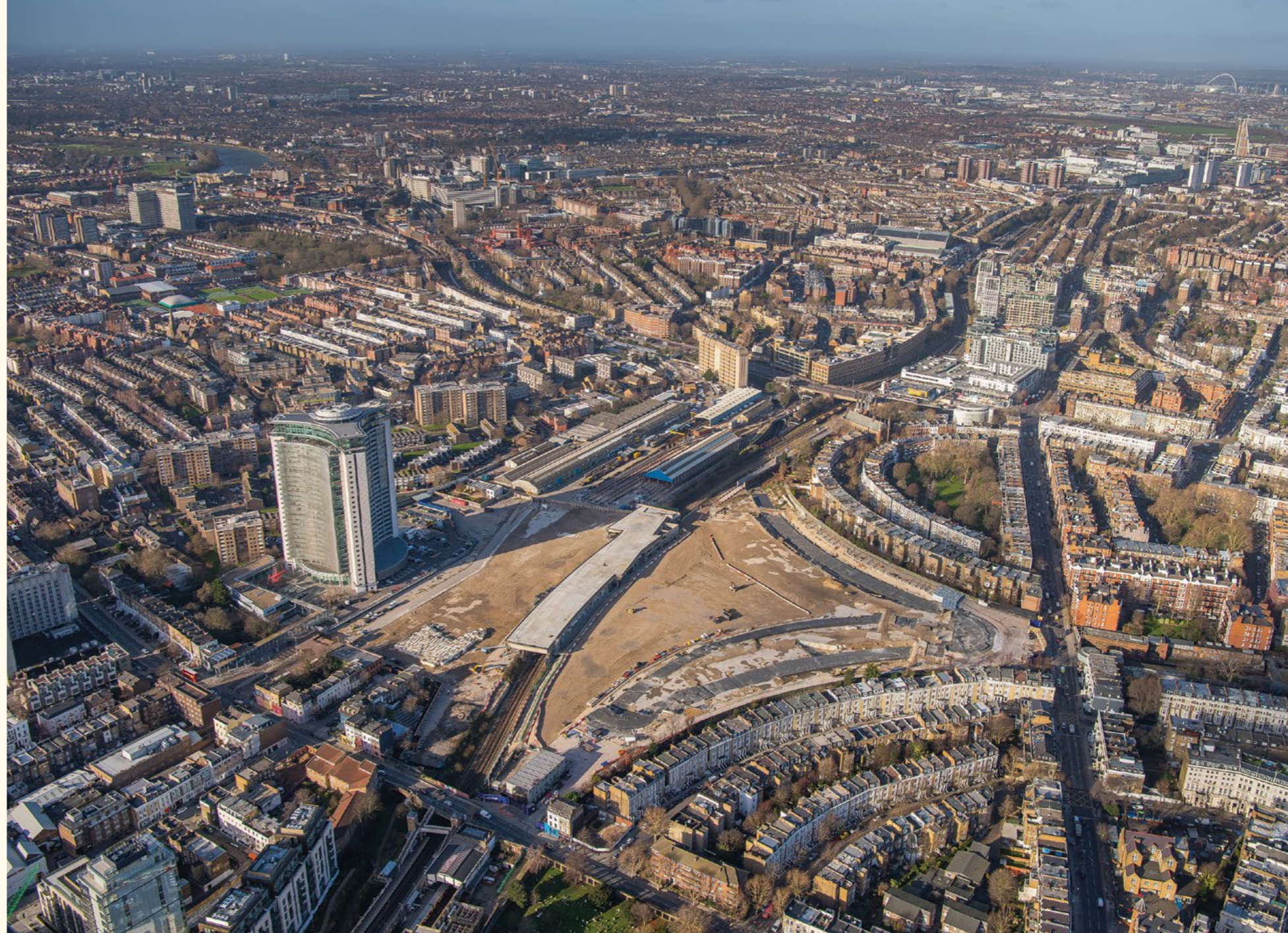
Above: Aerial image of the Earslough Site Right: Demolition of the Exhibition Centres
