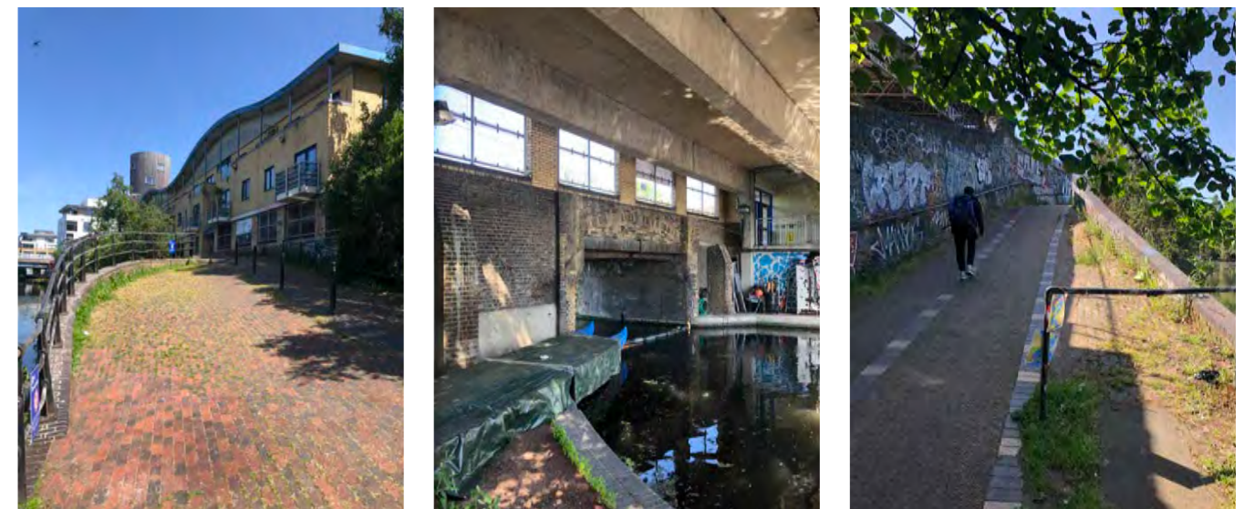
Fig 8.7: Photographs of the existing historic bridges along the Canal Towpath
