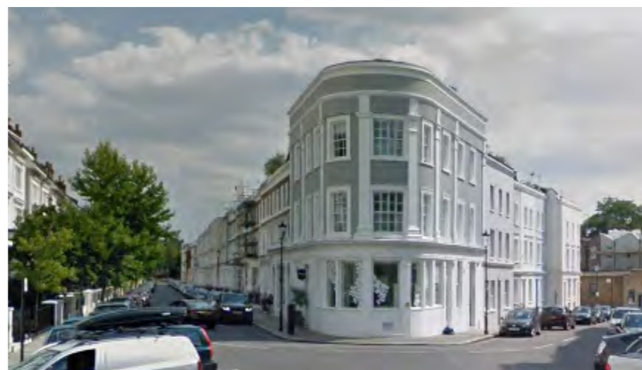
Fig 9.45: Regency frontages with definition to plinth
