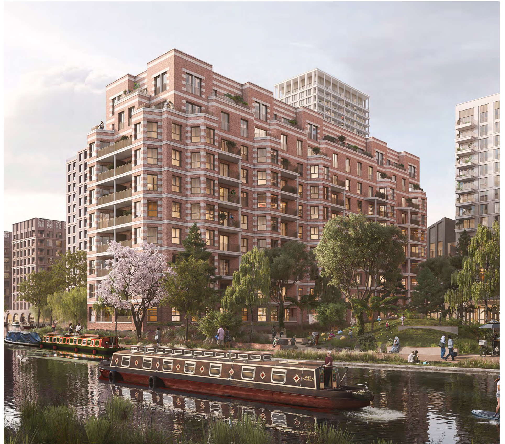
View looking East toward Building 4.4 from across the canal
