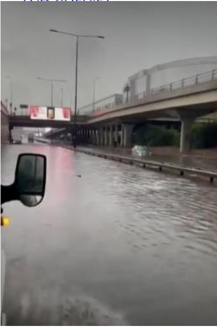
Figure 9-3: Roads acting as channels conveying floodwater. The images shown are the A3220, A40 and Portobello Road (images reproduced from the Standard 55 56 and Daily Mail 57 )
