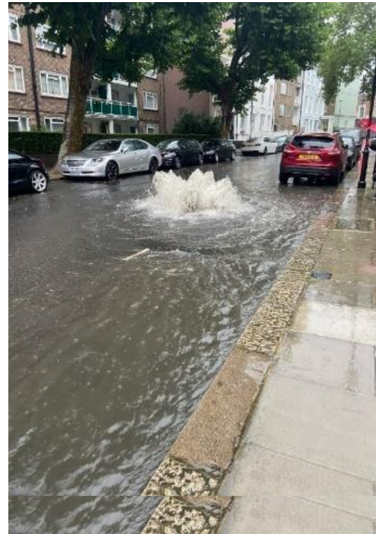
Figure 9-2: Fountains forming at manholes where the sewers are surcharged (images reproduced from a resident and i newspaper 54 ). Left: junction to St Marks Road and Lancaster Road; Right: Cornwall Crescent.
