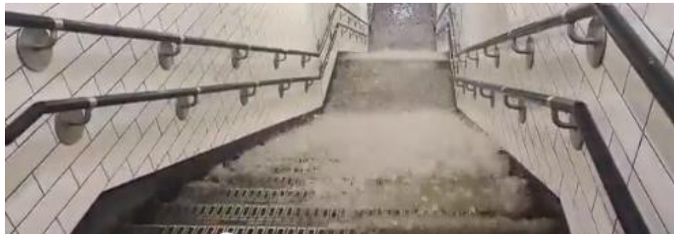
Figure 9-9: Flooding inside Sloane Square Station (image reproduced from Standard 59 ).
