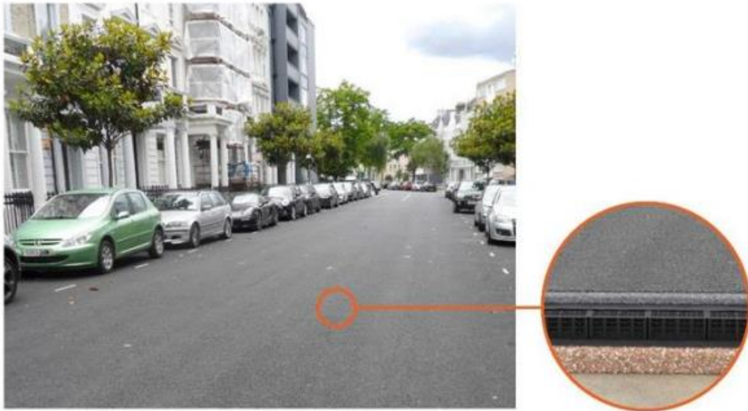
Figure 6-3: The SuDS scheme at Arundel Gardens showing the geocellular system underneath the road (image reproduced from Susdrain 42 ).
