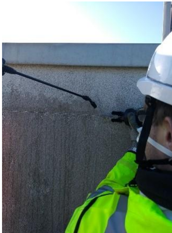
Image of the process and water suppression
