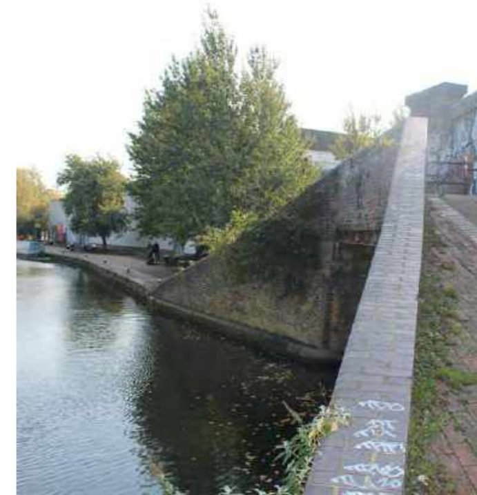
Fig 3.9: The existing bridge over the former canal basin
