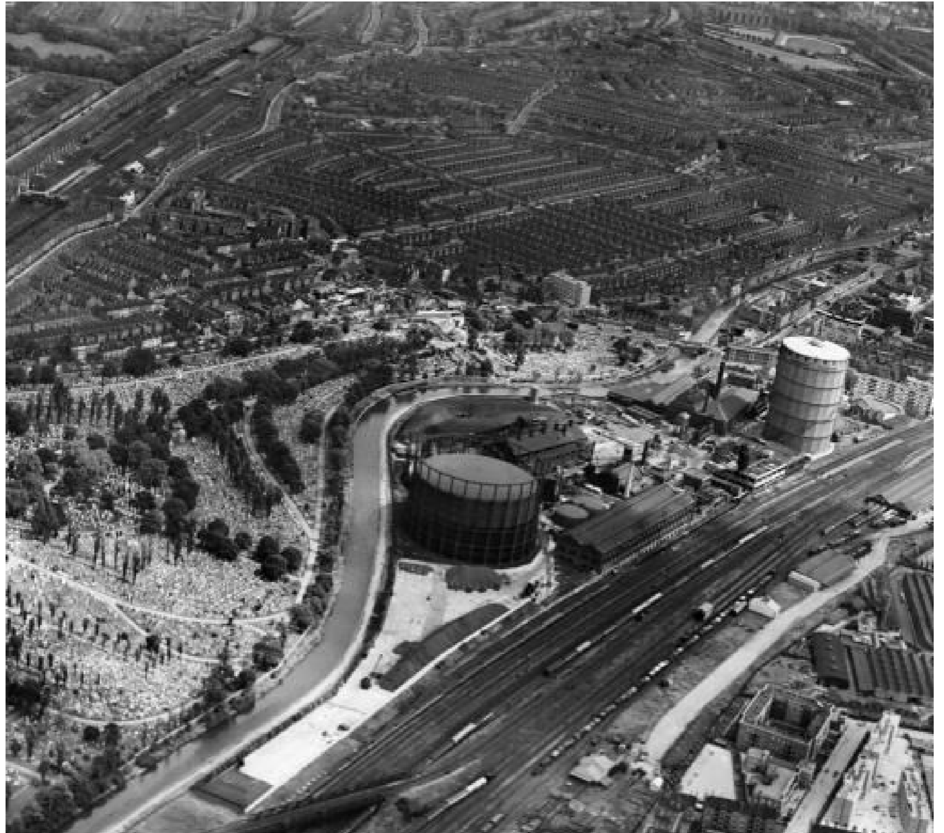
Fig 3.17: Aerial view of former Gas Works site viewed from the west
