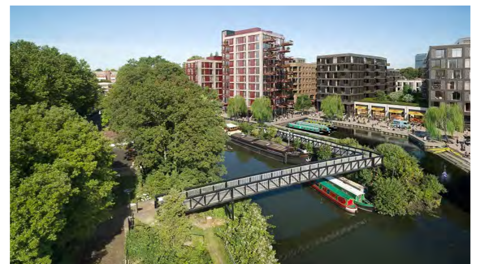
Fig 1.3: The Brentford Project
