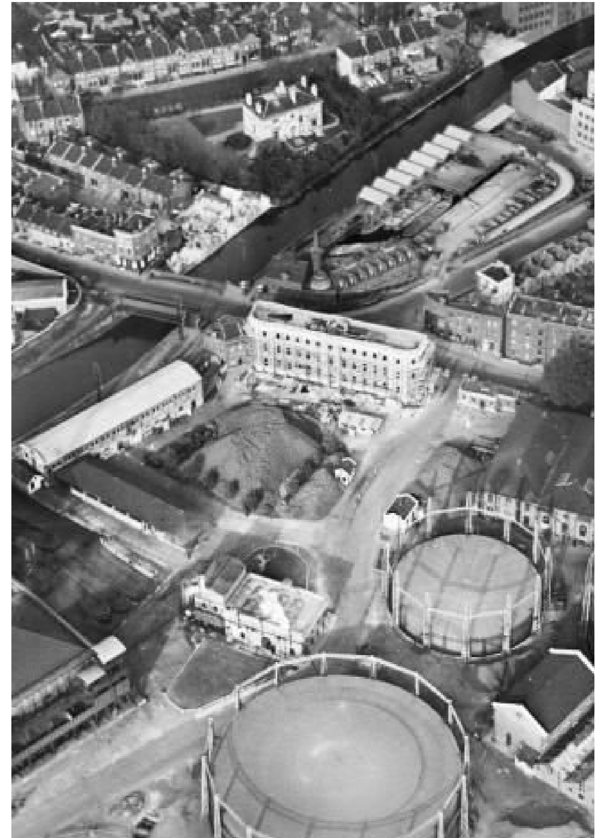
Fig 3.19: The site, prior to the construction of Kensal House
