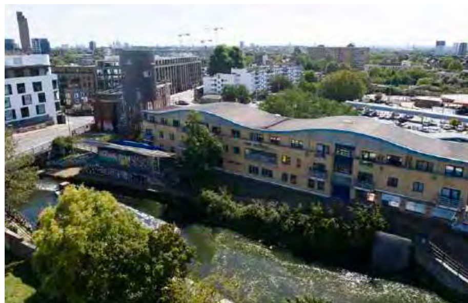
Fig 3.118: An aerial view of the Boathouse Centre taken in August 2023.
