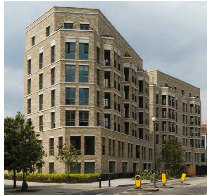
South Gardens, Elephant & Castle, Maccreeanor Lavington Architects
