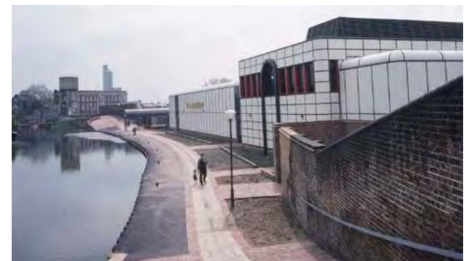
Fig 3.76: Point 1: The existing store, shortly after opening in 1988.
