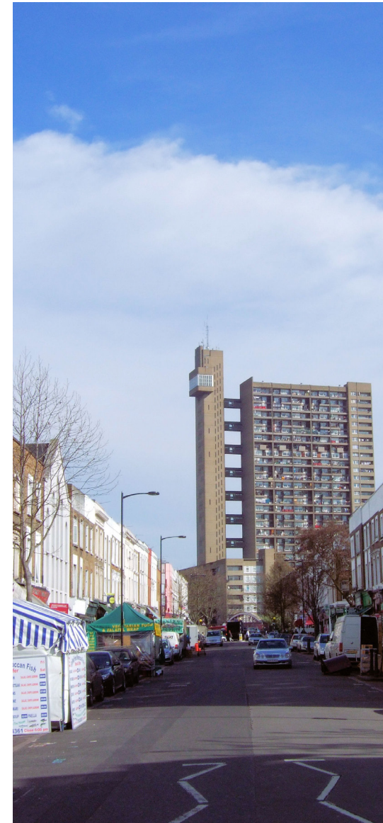
Trellick Tower from Golborne Road © Jim Linwood / Flickr
